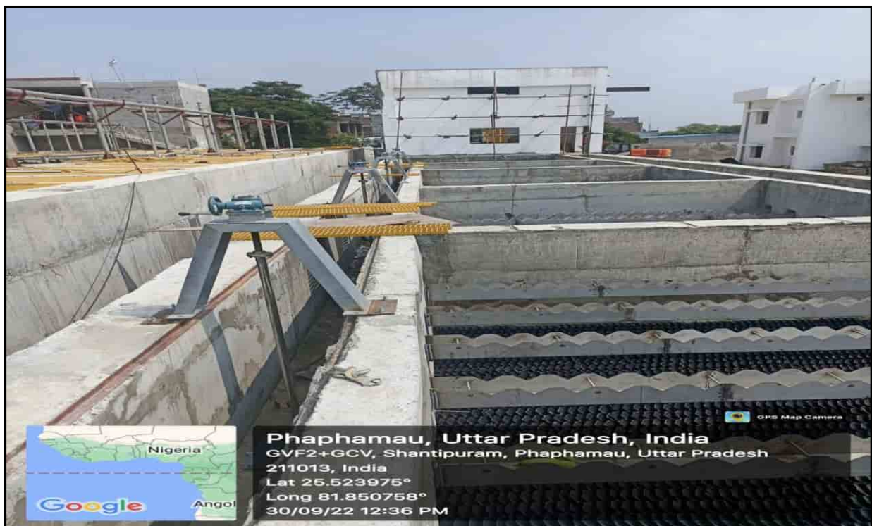
Tube Settler (STP) – E&M work under progress
