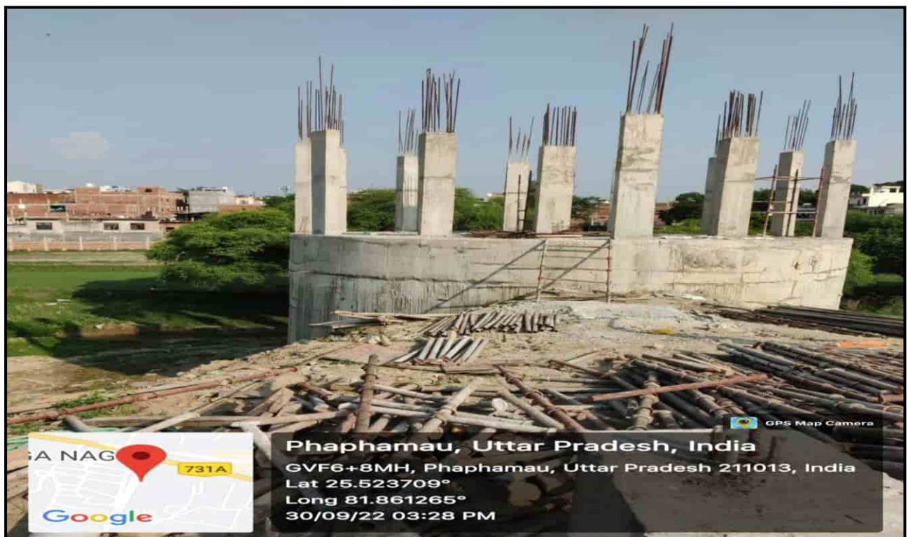
Basna Nalla SPS: Column casting work in progress
