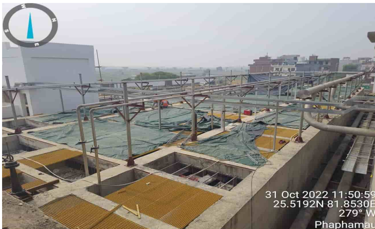
FCR (STP): E&M work under progress for FCR module
