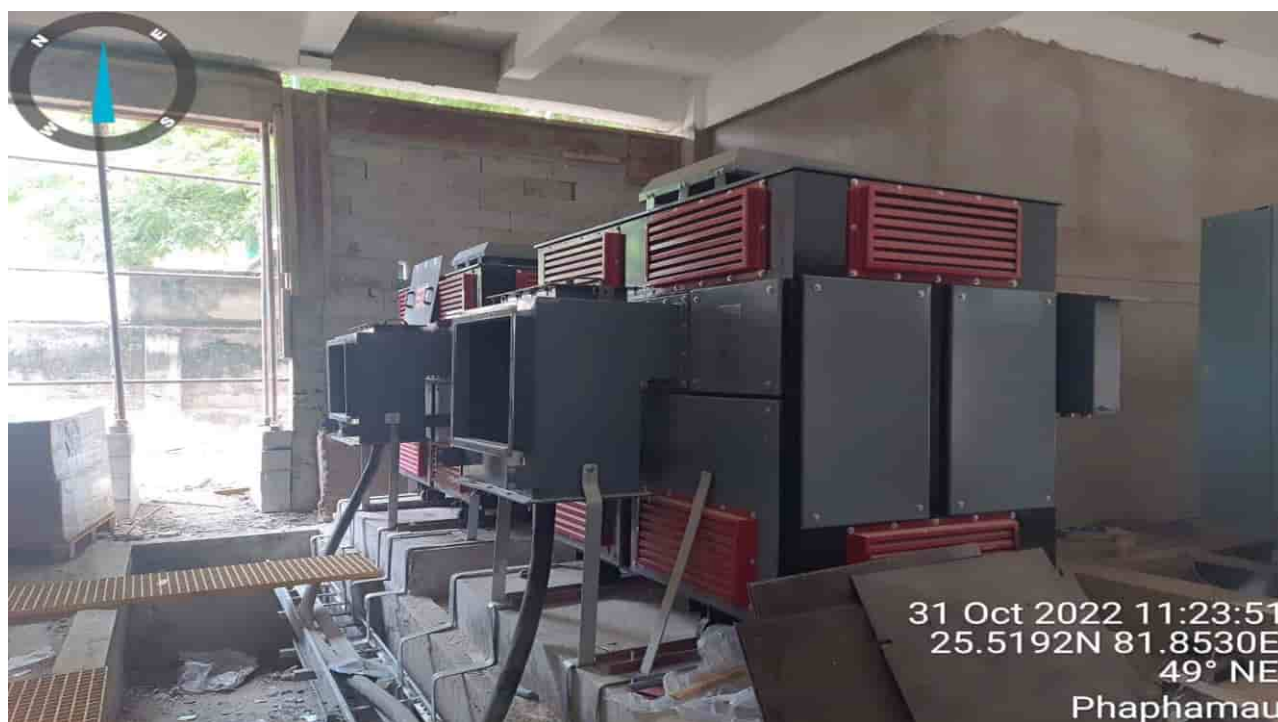
Process Building (STP) – Transformer erection work under progress
