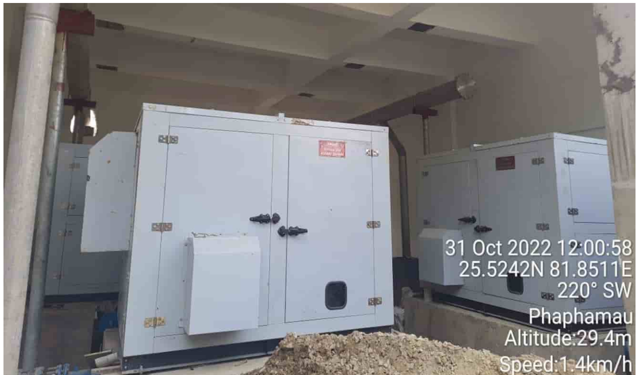
Process Building (STP) – FCR Air blower erection work under progress
