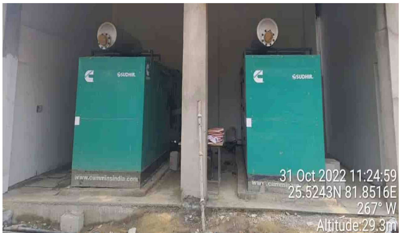
Process Building (STP) – DG erection work under progress
