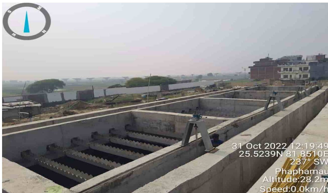
Tube Settler (STP) – E&M work under progress
