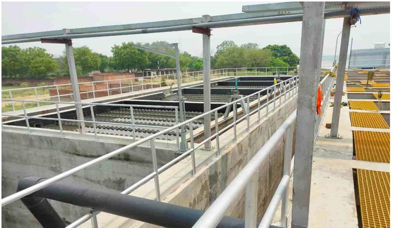
Tube settler– Current Status (Functional)
