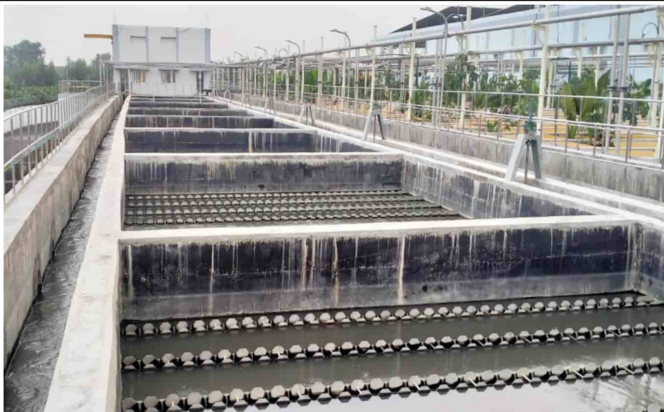
Tube settler– Current status (Functional)
