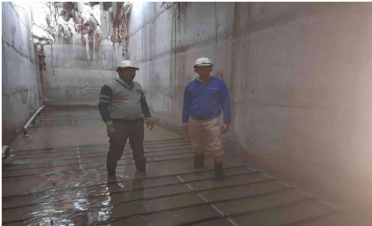
FCR (STP): Diffuser installation under progress
