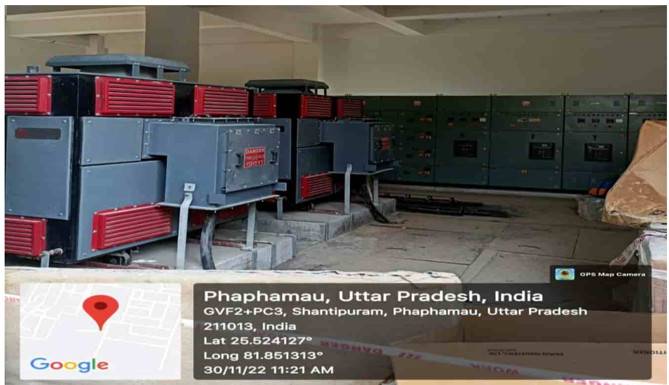
Process Building (STP) – Transformer & HT panel charging completed
