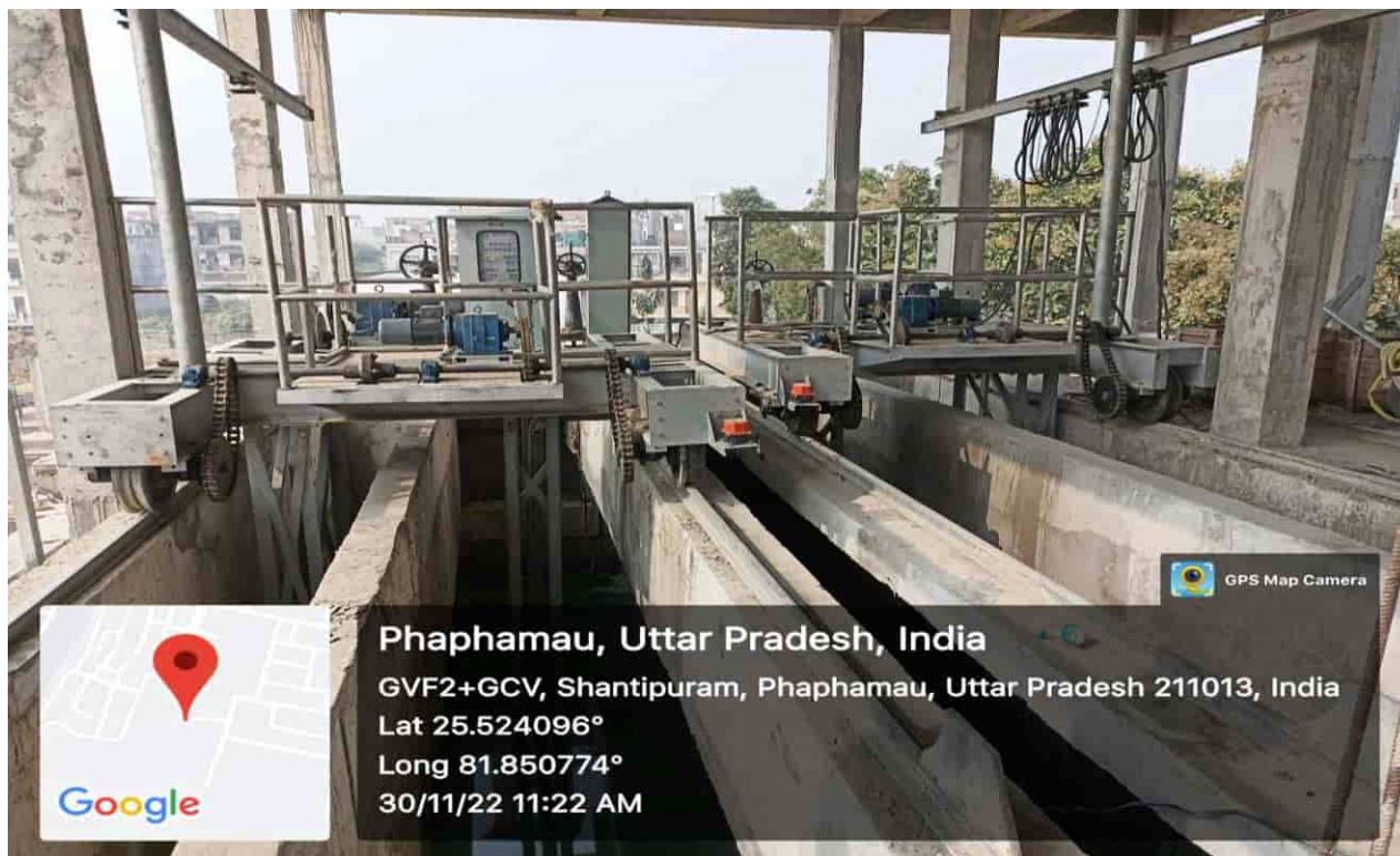
Process Building (PTU) – Grit Mechanism erection work as well as civil finishing work under progress
