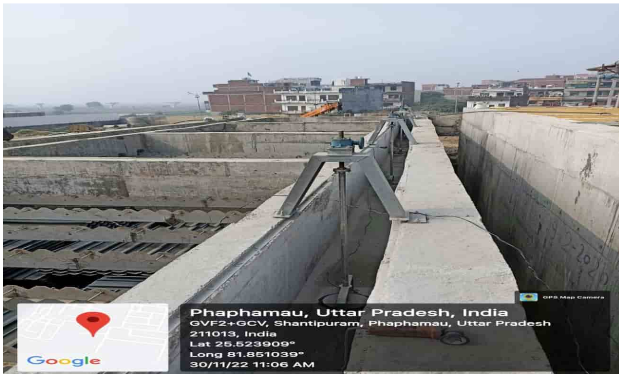
Tube Settler (STP) – Hydro testing under progress
