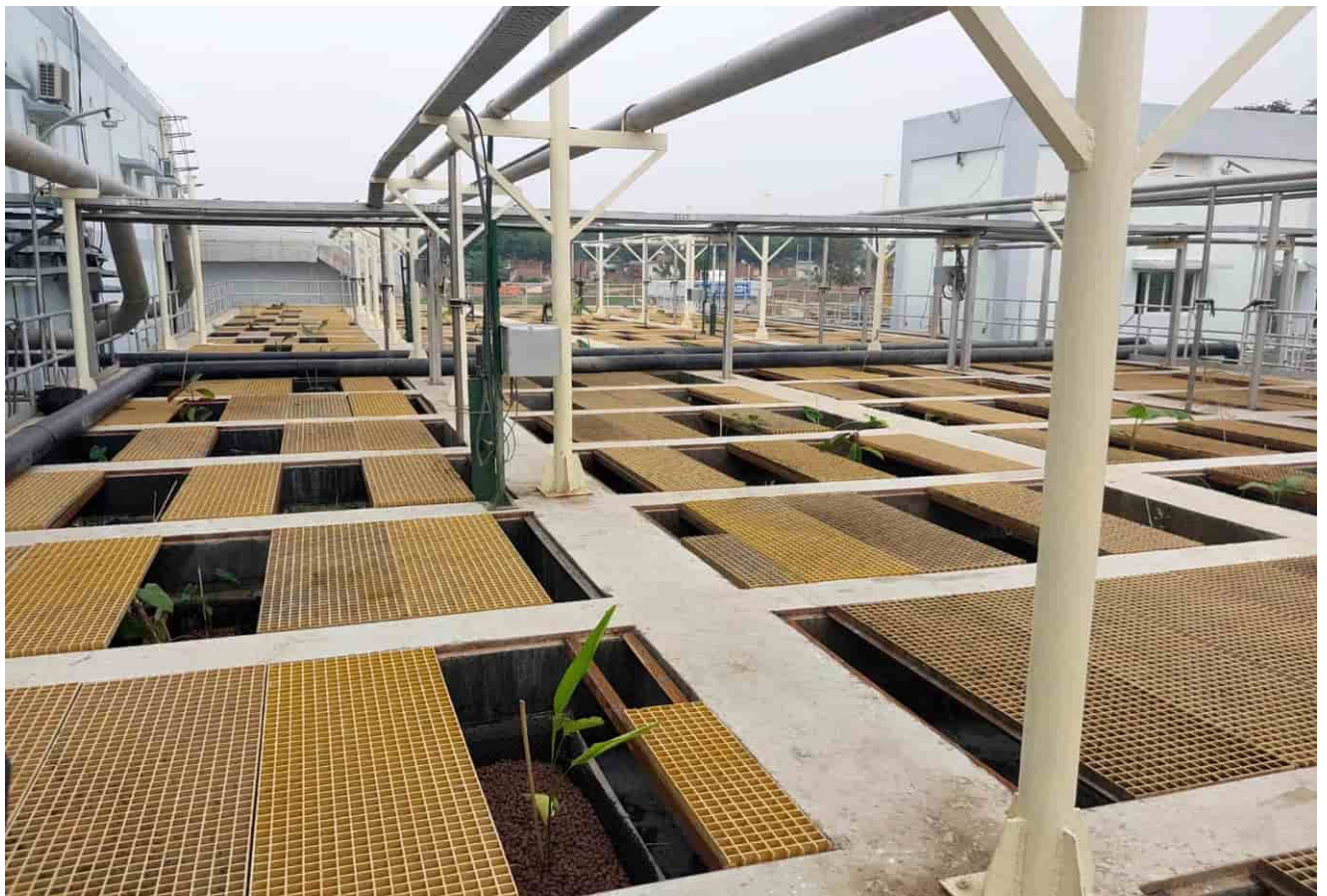
Tube settler– Current Status (Functional)
