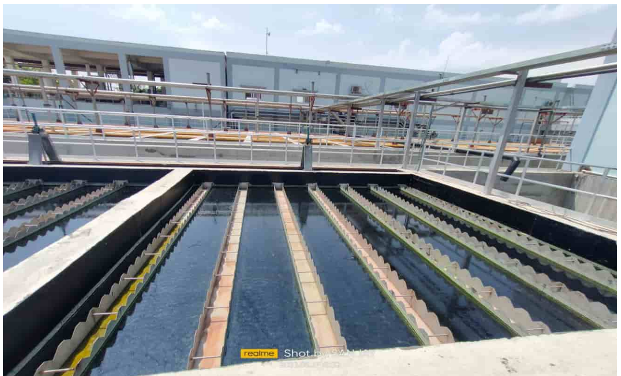
Tube settler– E&M work under progress
