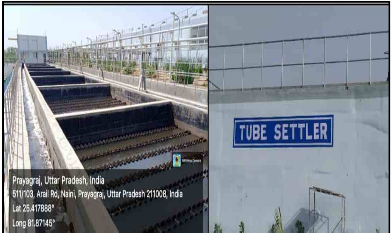
Tube settler- Current status (Functional)
