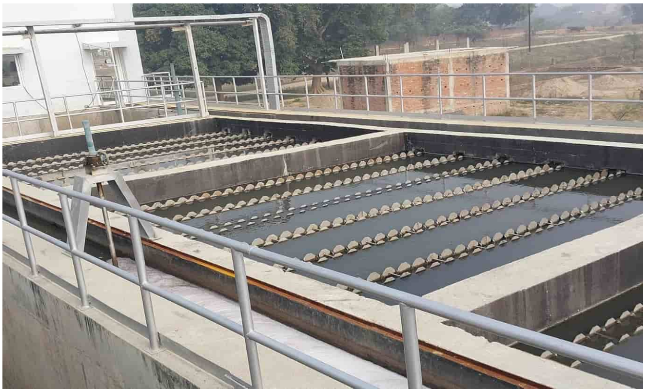
Tube settler– Current Status (Functional)
