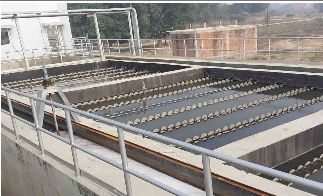
Tube settler– Current Status (Functional)
