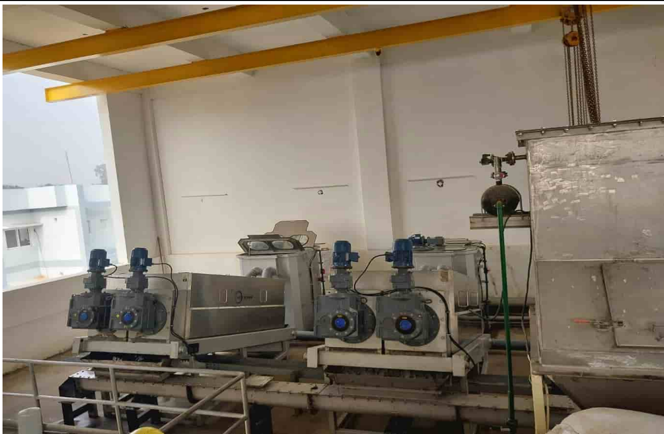
Sludge Dewatering Unit – Current status (Functional)
