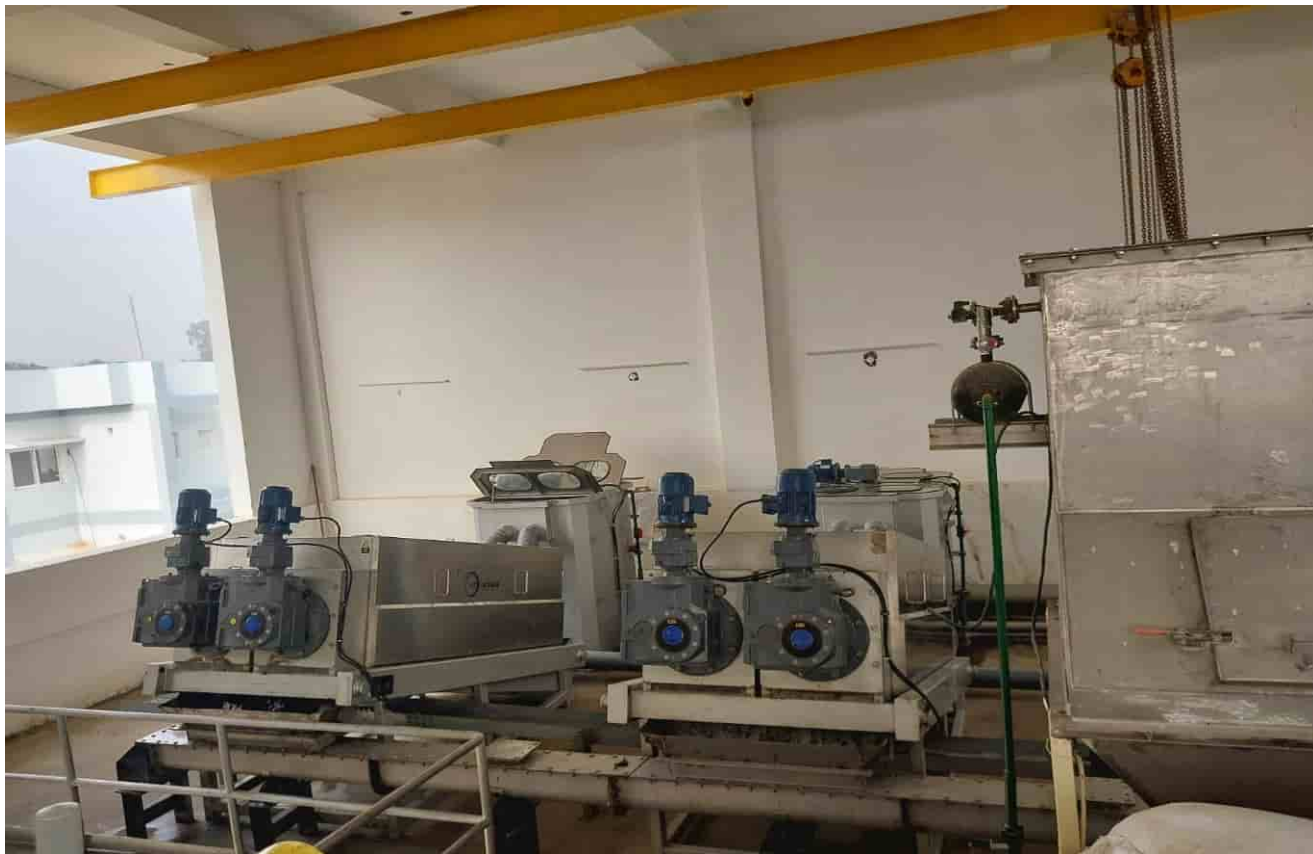
Sludge Dewatering Unit – Current status (Functional)
