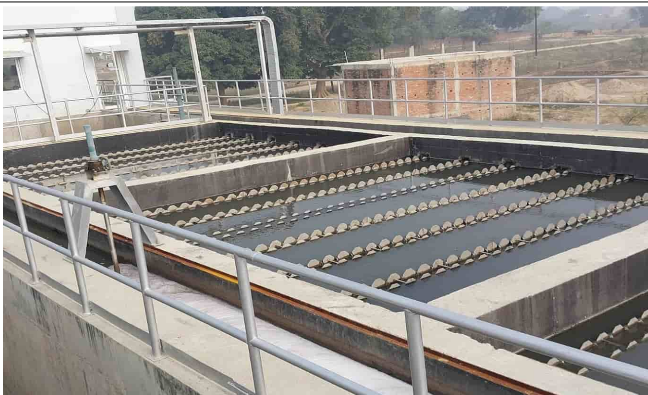
Tube settler– Current Status (Functional)
