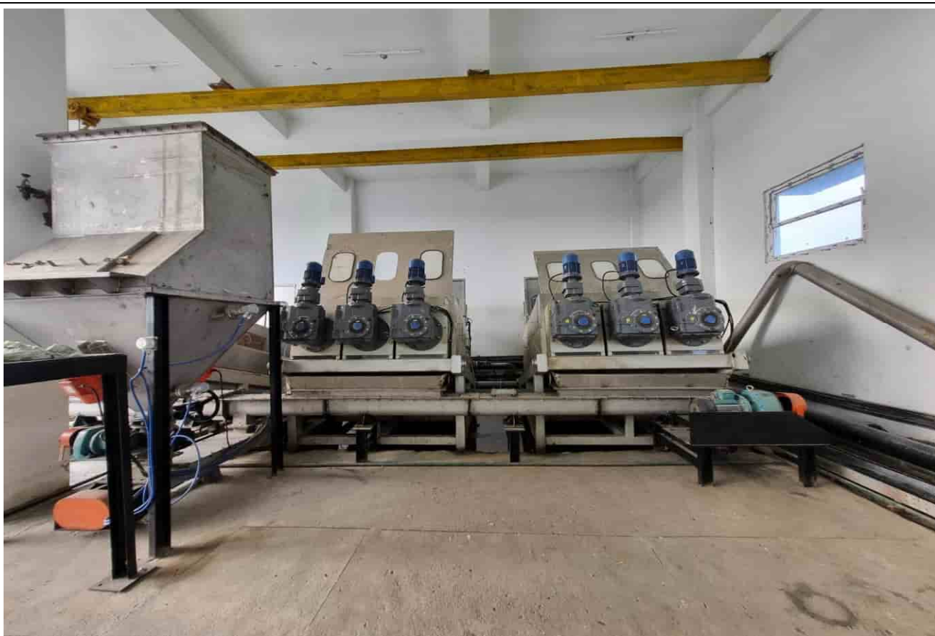
Sludge Dewatering Unit – Current status (Functional)
