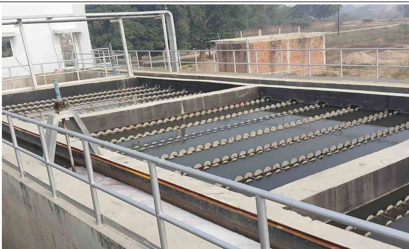
Tube settler– Current Status (Functional)
