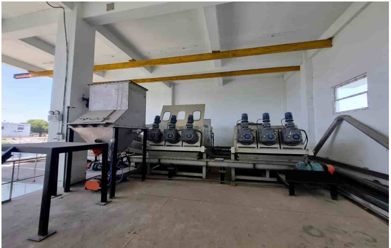
Sludge Dewatering Unit – Current status (Functional)
