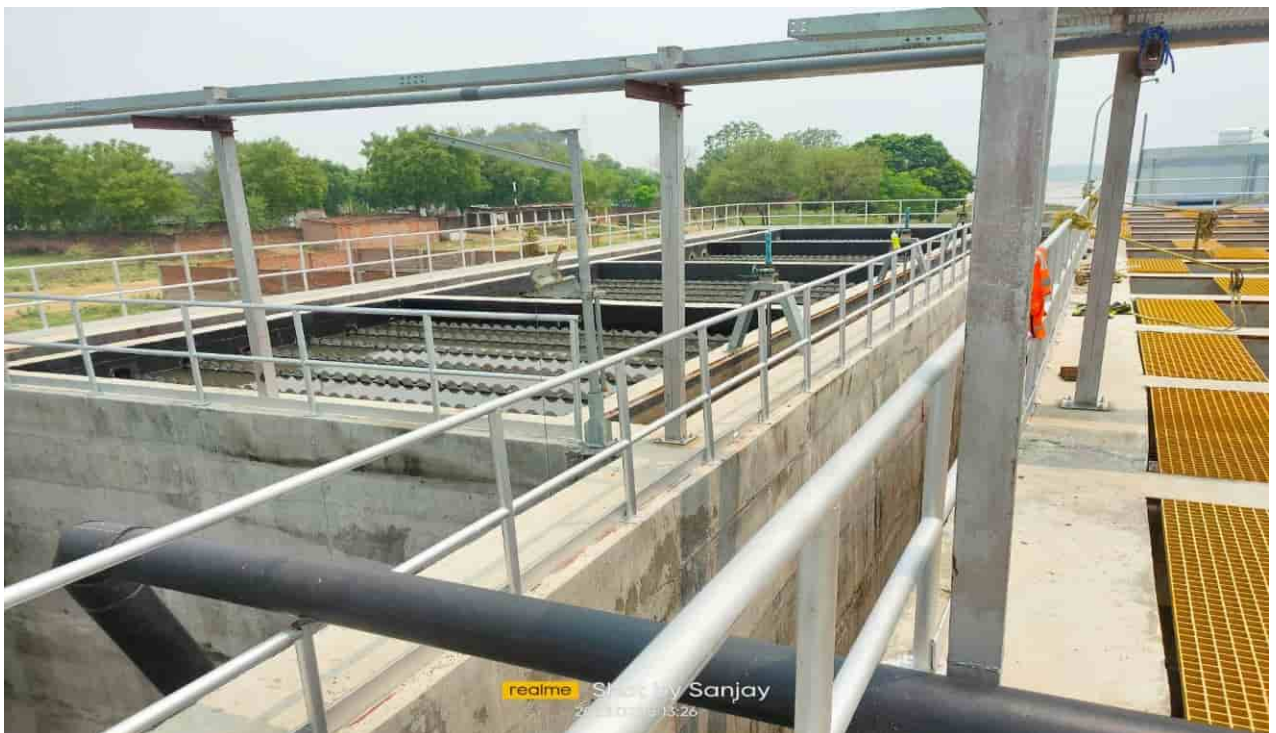
Tube settler– Current Status (Functional)
