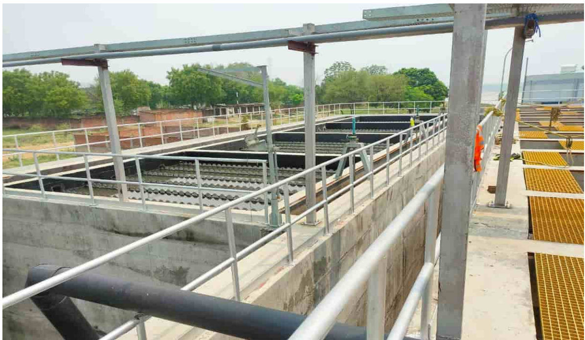
Tube settler– Current Status (Functional)
