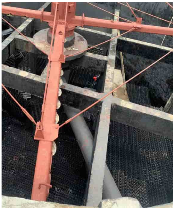
Bio Tower – Media replacing work
