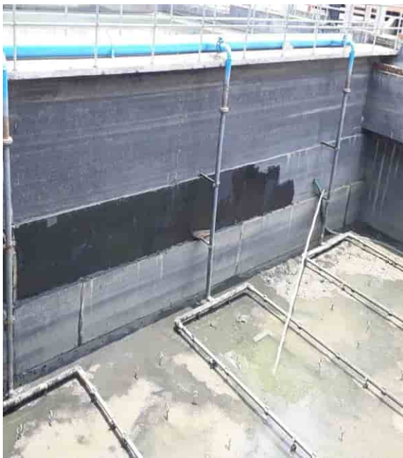
Aeration Tank - Epoxy paint on wall
