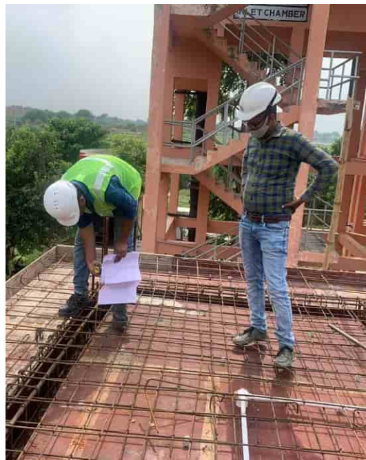
PLC Room – Reinforcement of slab checked by Aecom Engineer
