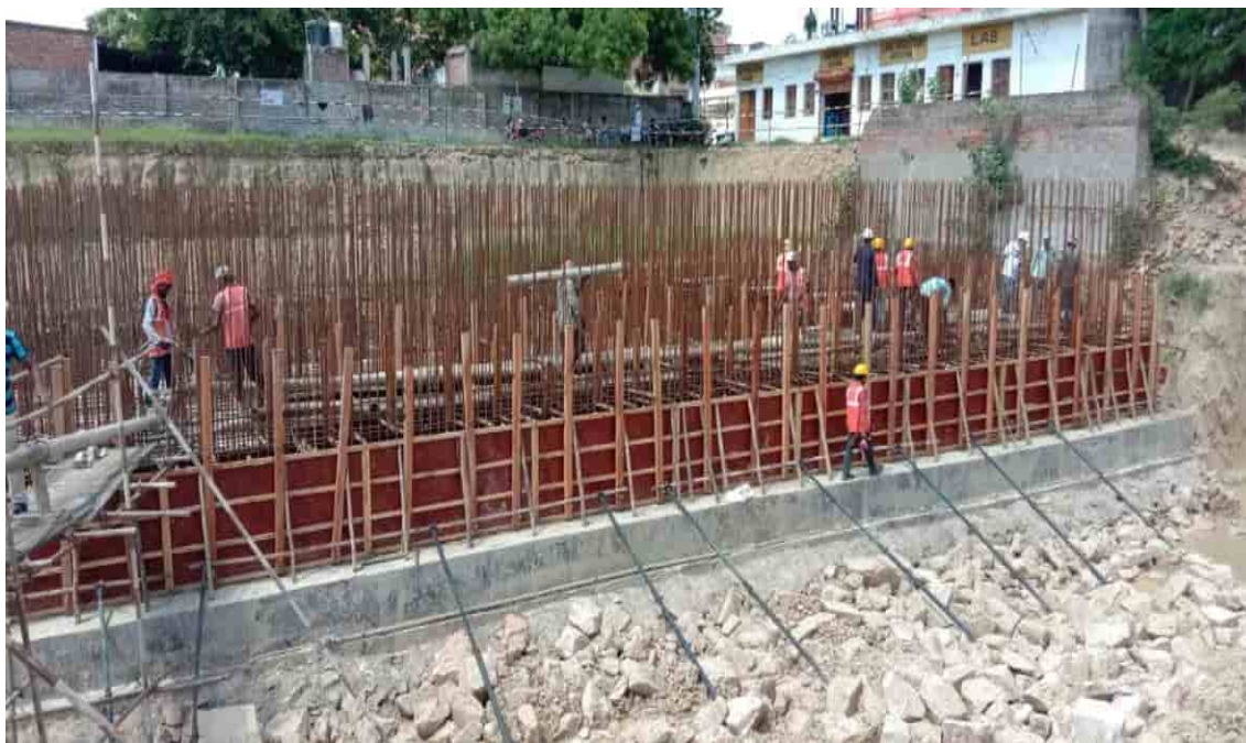
FCR – Wall shuttering work
