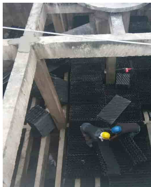
Bio Tower – Media replacing work
