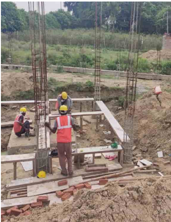
Staff Quarter – Plint beam shuttering work
