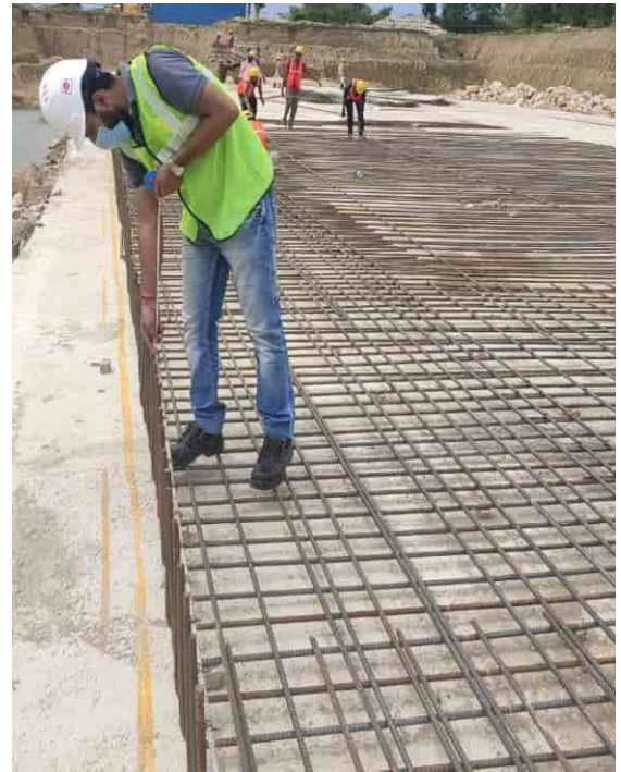
FCR –Reinforcement of bottom raft checked by Aecom Engineer
