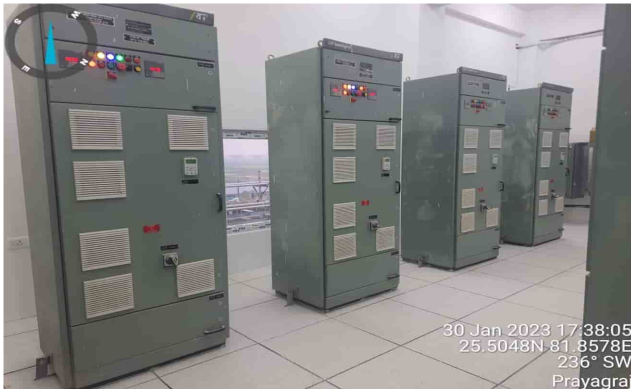
Process Building (STP) – Panel erection work completed
