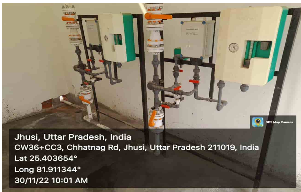
Process Building (Chlorination room)– Chlorination work is under progress
