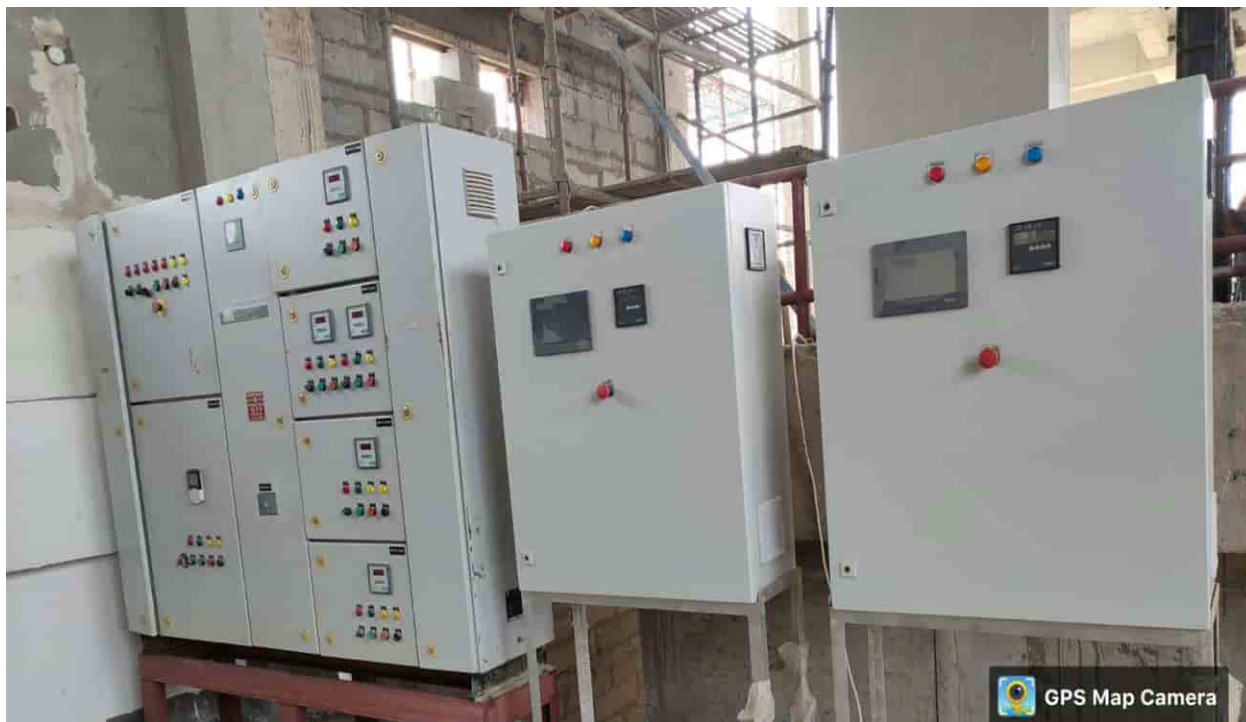
Process Building – LCP erection work is under progress
