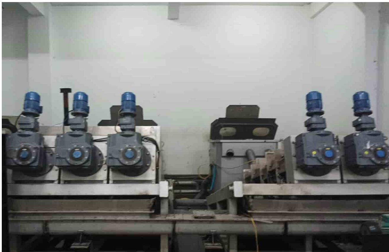
Sludge Dewatering Unit – Current status (Functional)
