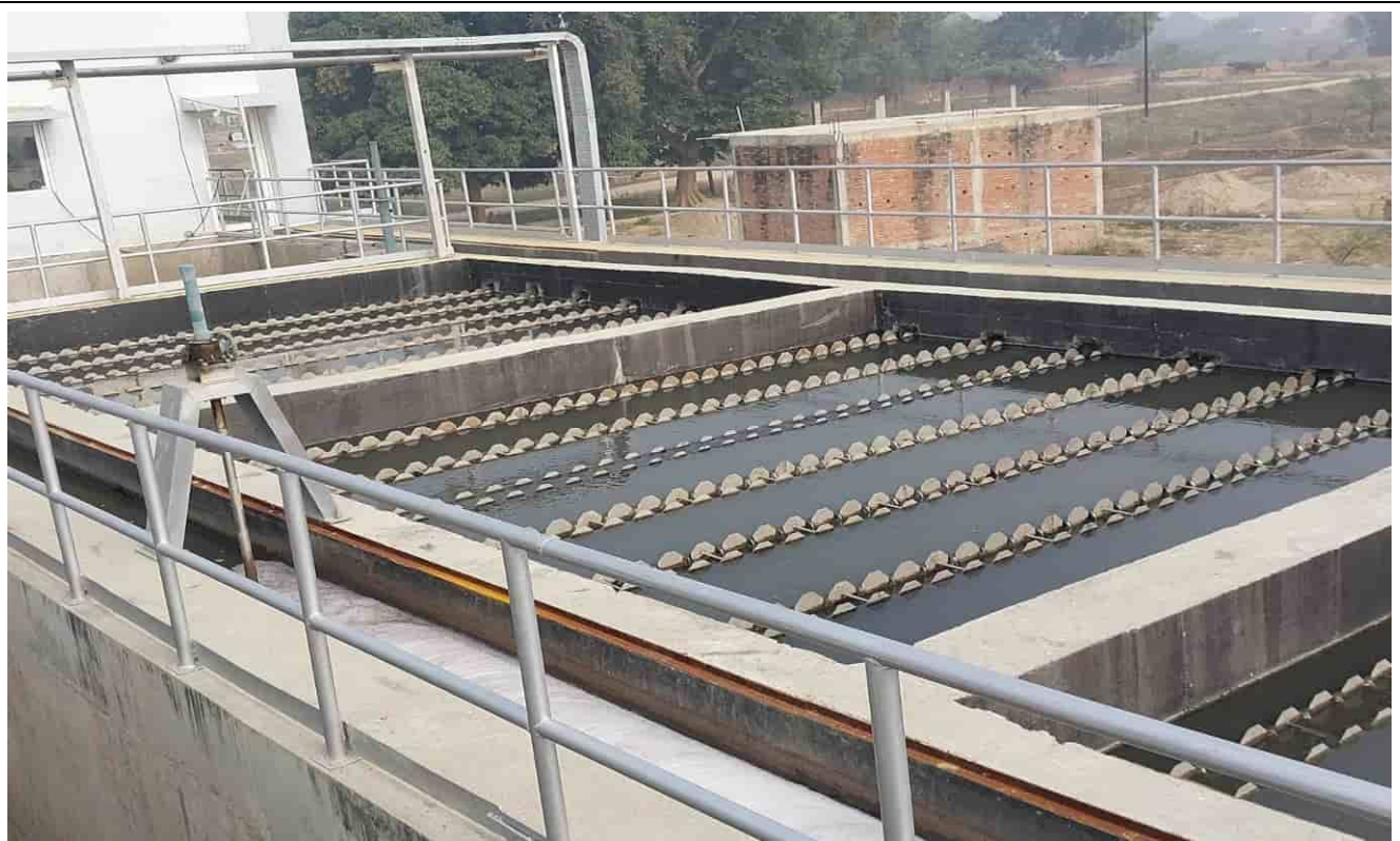
Tube settler– Current Status (Functional)
