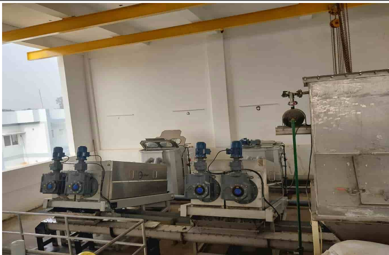
Sludge Dewatering Unit – Current status (Functional)
