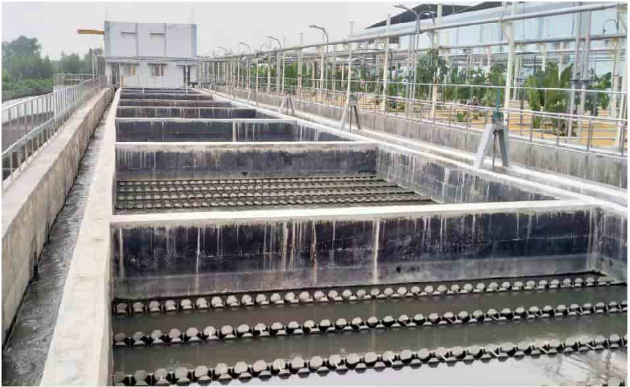
Tube settler– Current status (Functional)
