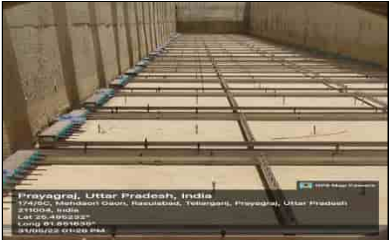
FCR (STP): Diffuser grid frame Erection work under progress
