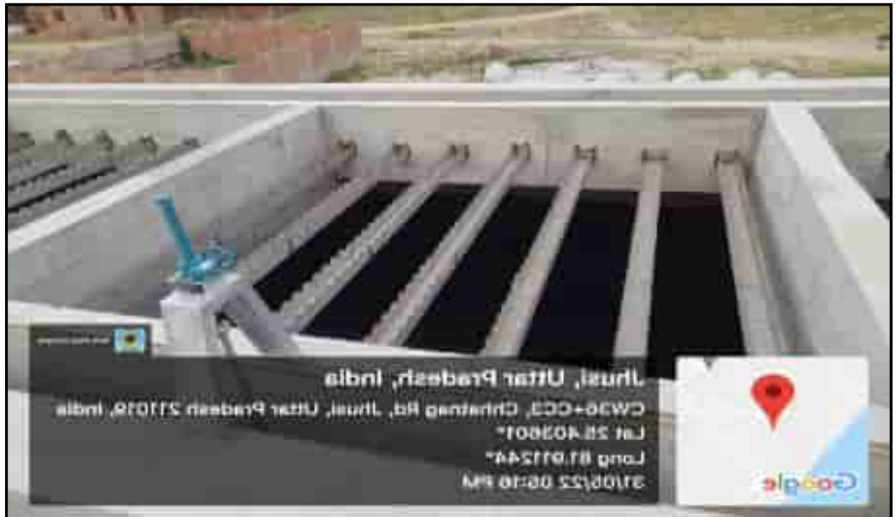
Tube settler – Poppet valve and Launder erection work under progress
