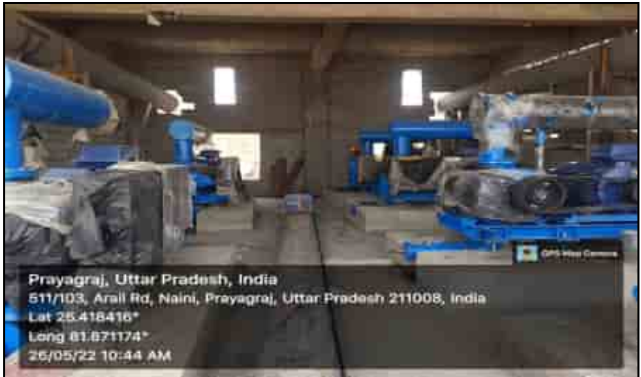
FCR (STP) – Air Blower erection work under progress
