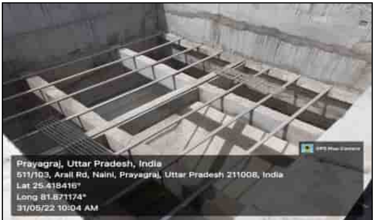
Tube settler (STP) – Support base frame erection work under progress
