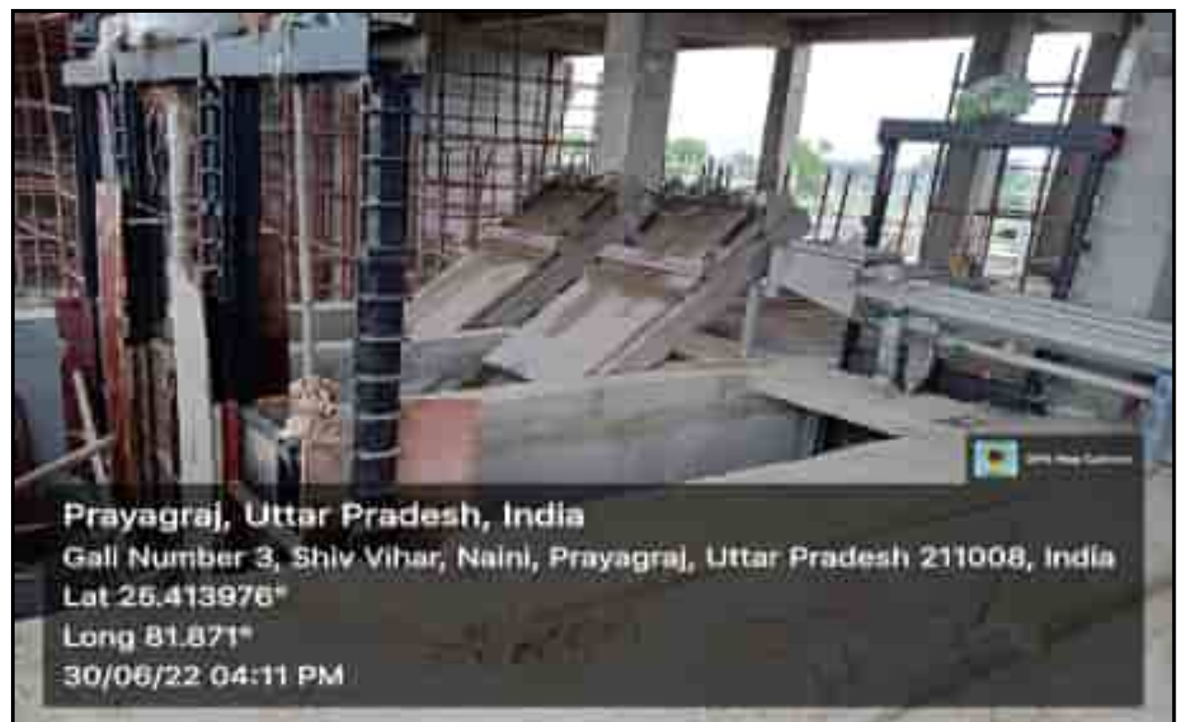
Process building (PTU) – Screen erection work under progress
