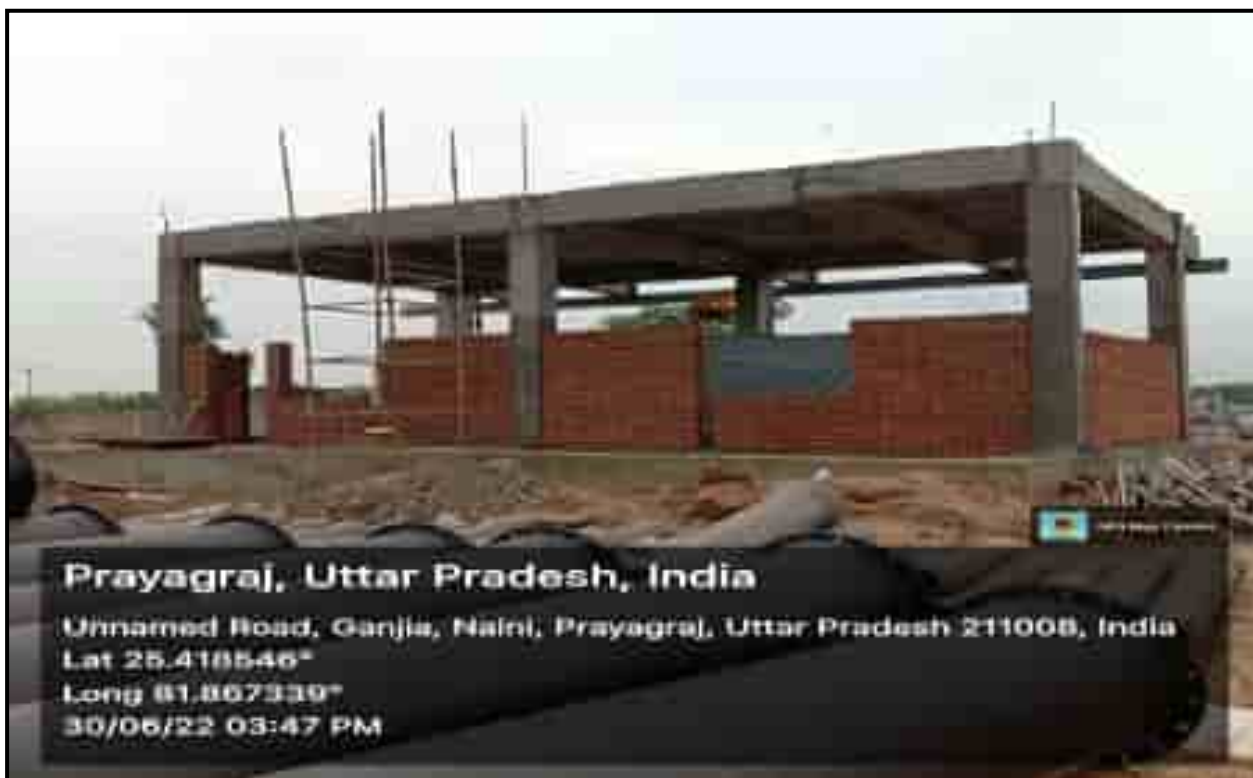
Naini-II MPS (Panel room)– Brick work under progress
