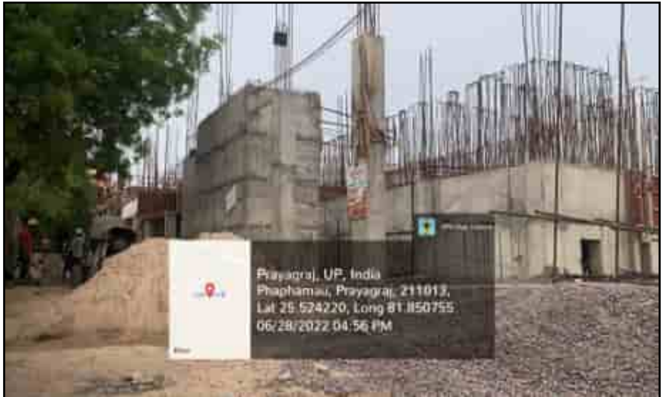
Process Building (STP) – Column casting work under progress
