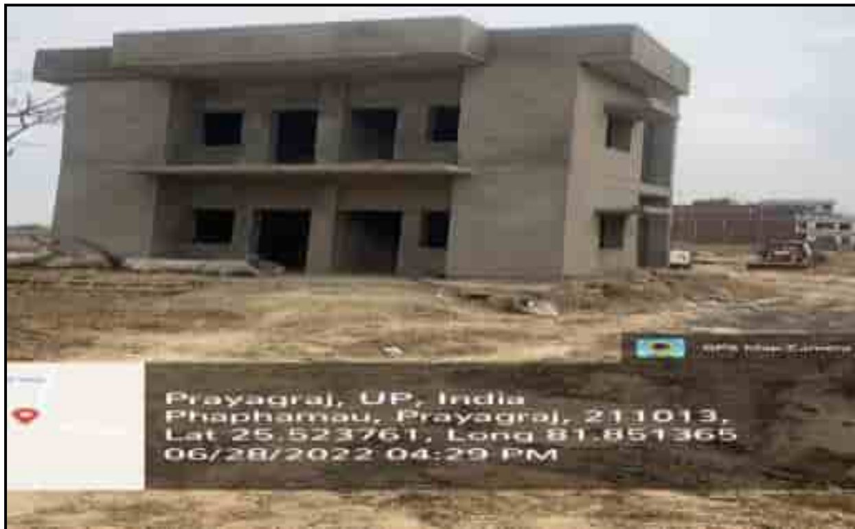
Staff Quarter (STP)– Plastering work completed
