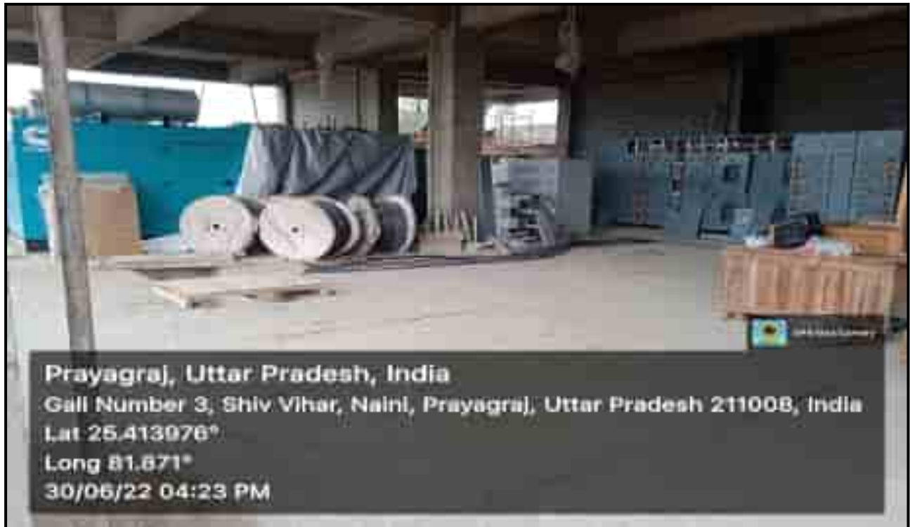
Process Building (DG and Panel room) –DG and Panel erection work under progress
