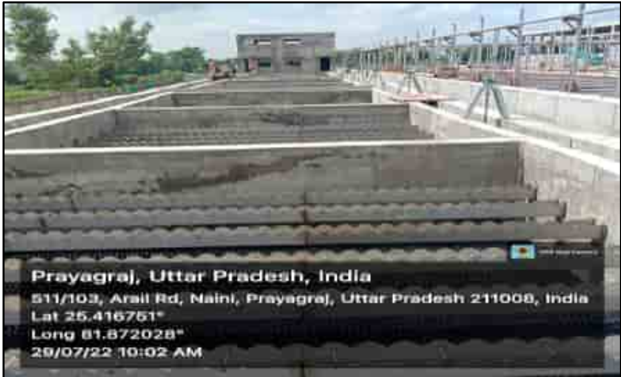
Tube settler – Mechanical work under progress
