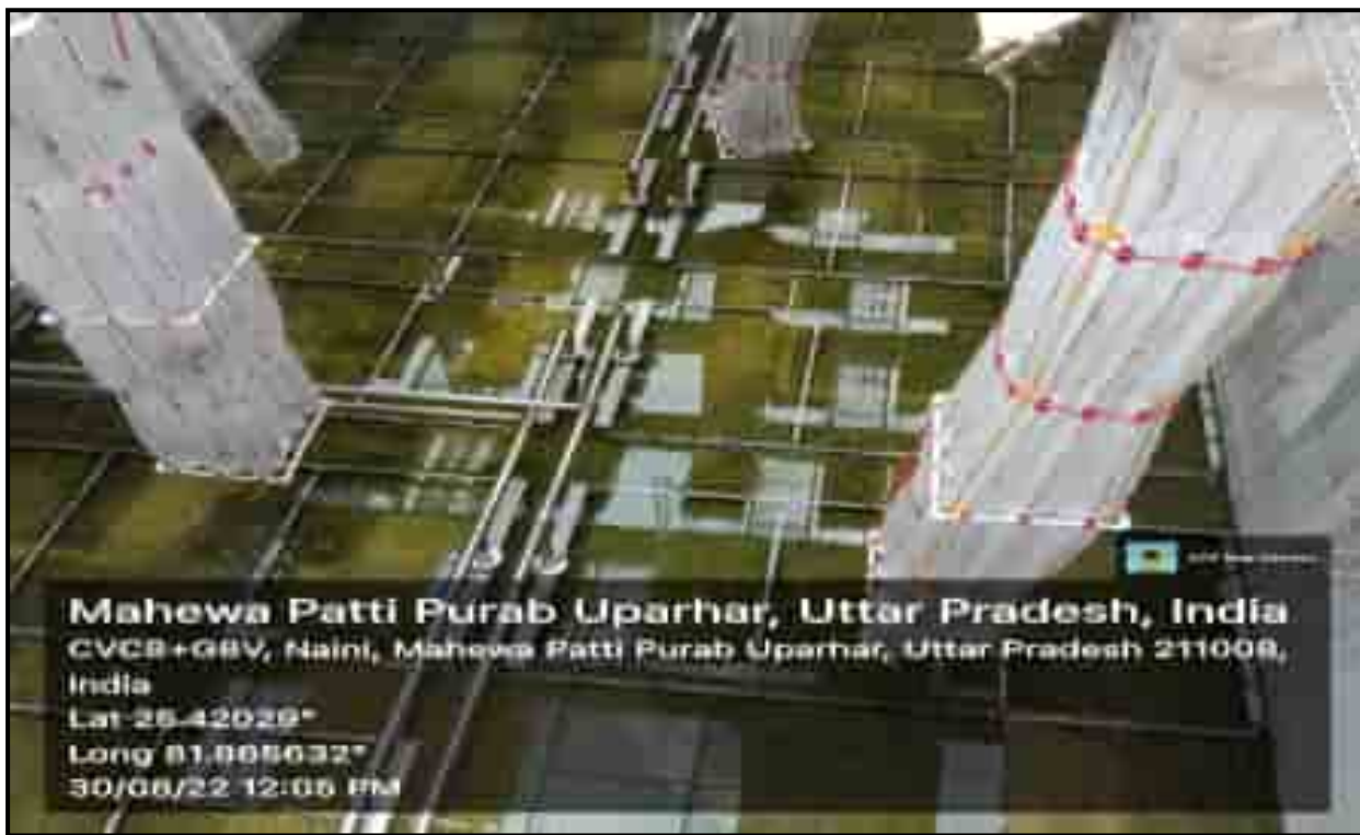
FCR – E&M (Air diffuser grid piping) work under progress
