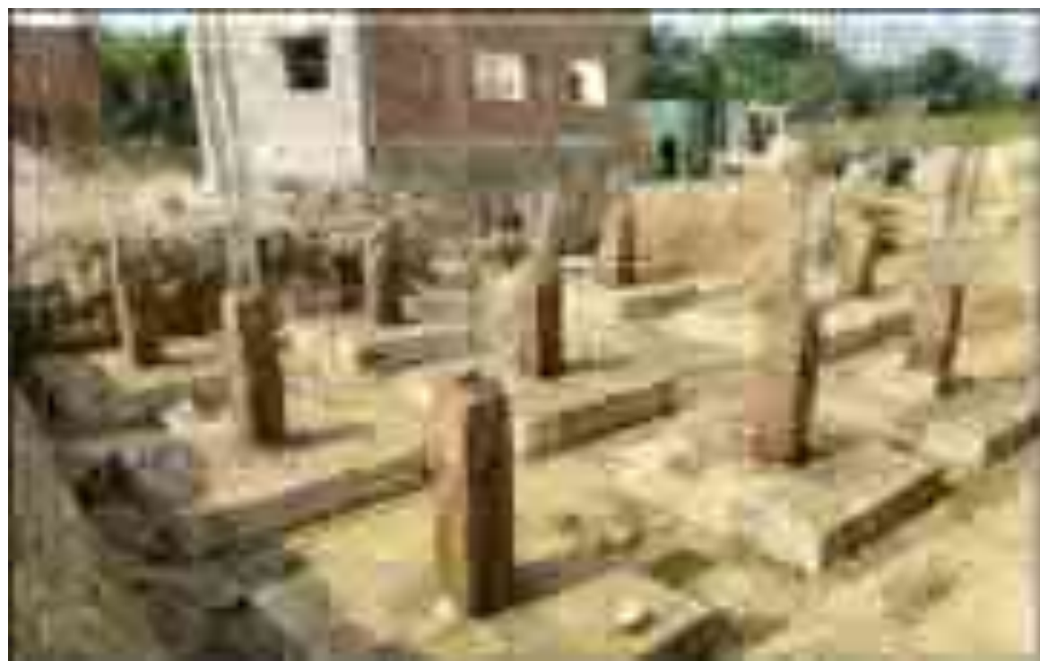
Staff Quarter – RCC of column above footing work in progress
