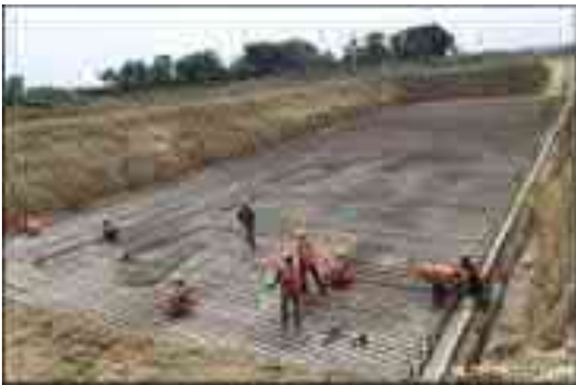
FCR tank – Reinforcement laying and binding work in progress
