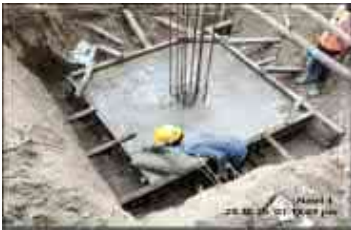
Compressor building – Casting of footing work in progress
