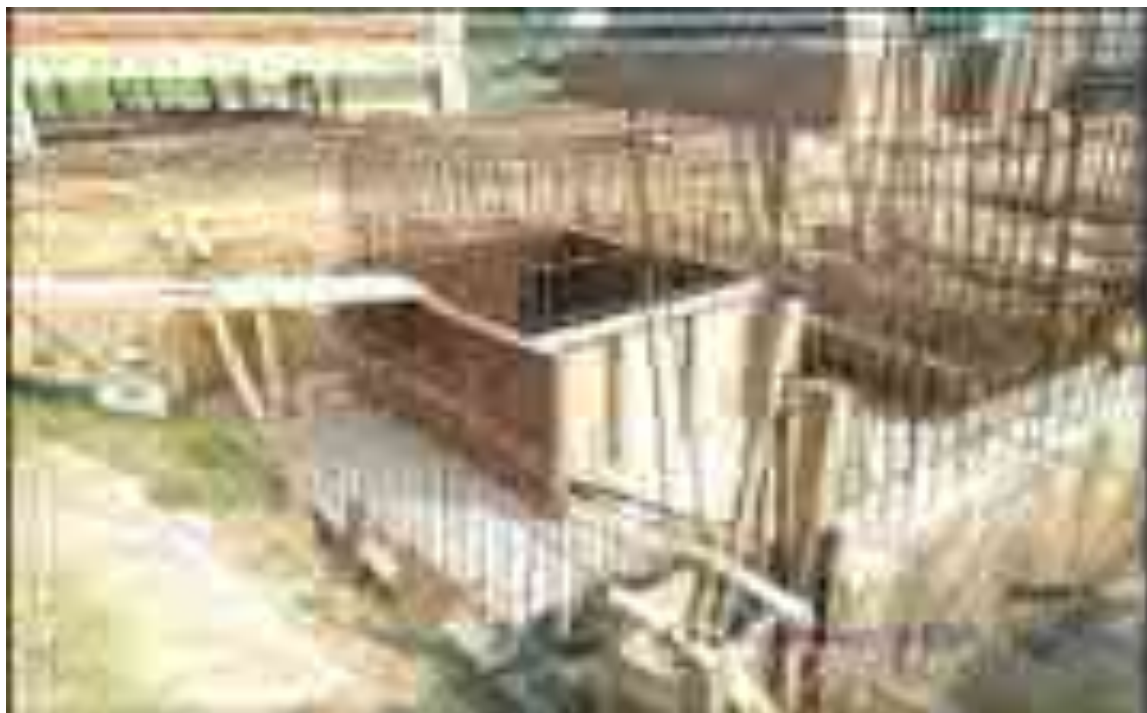
Transformer foundation - Shuttering work in progress
