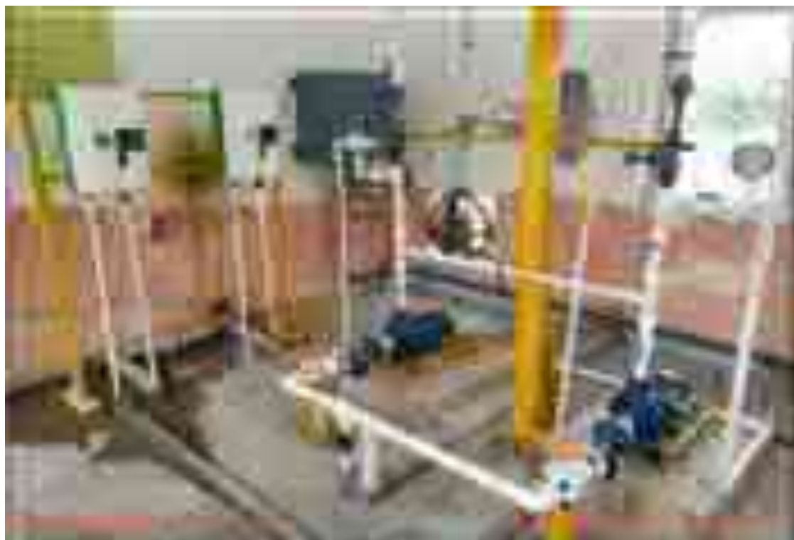
Chlorinator system in under operation
