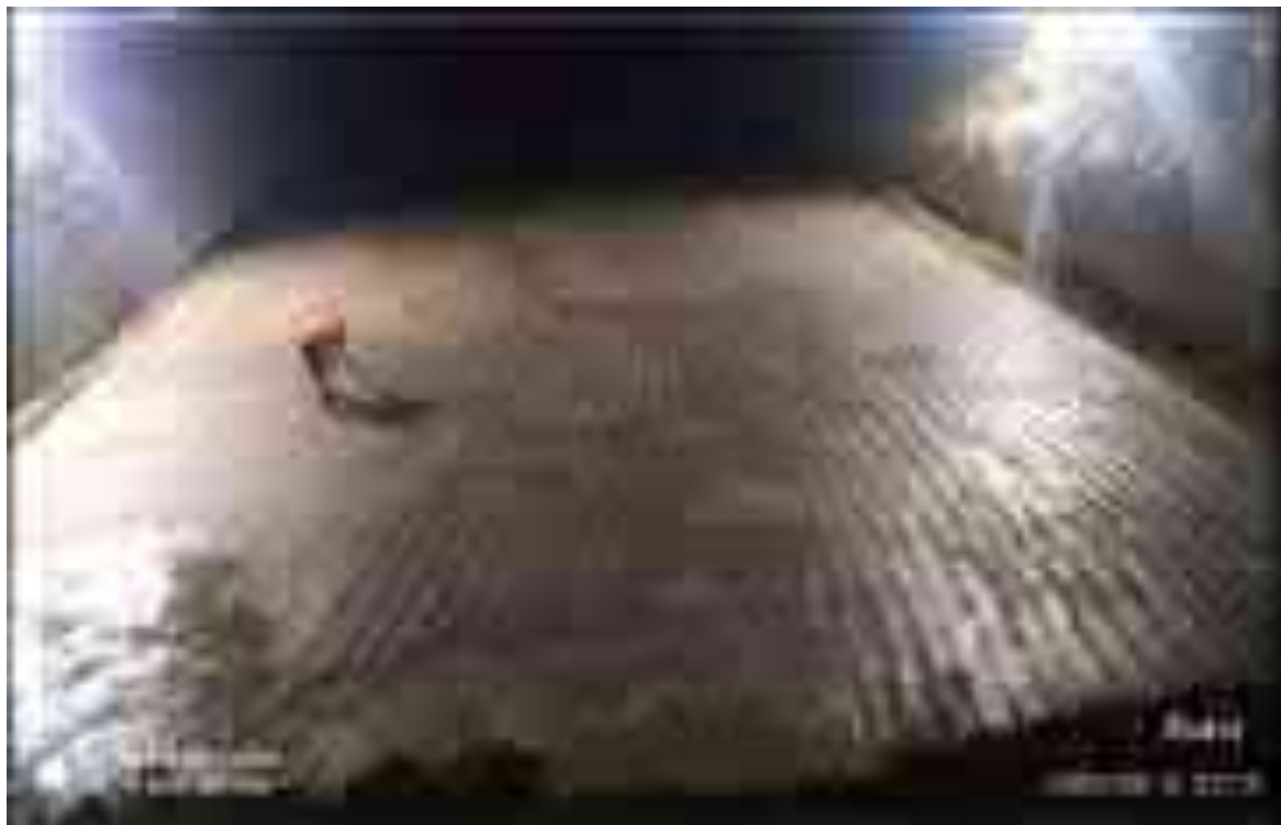
FCR tank – PCC work completed
