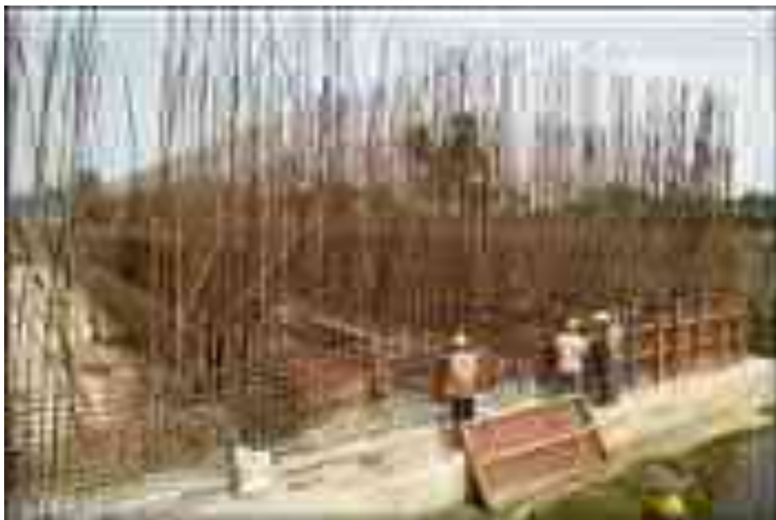
FCR tank – Lift wall shuttering work in progress
