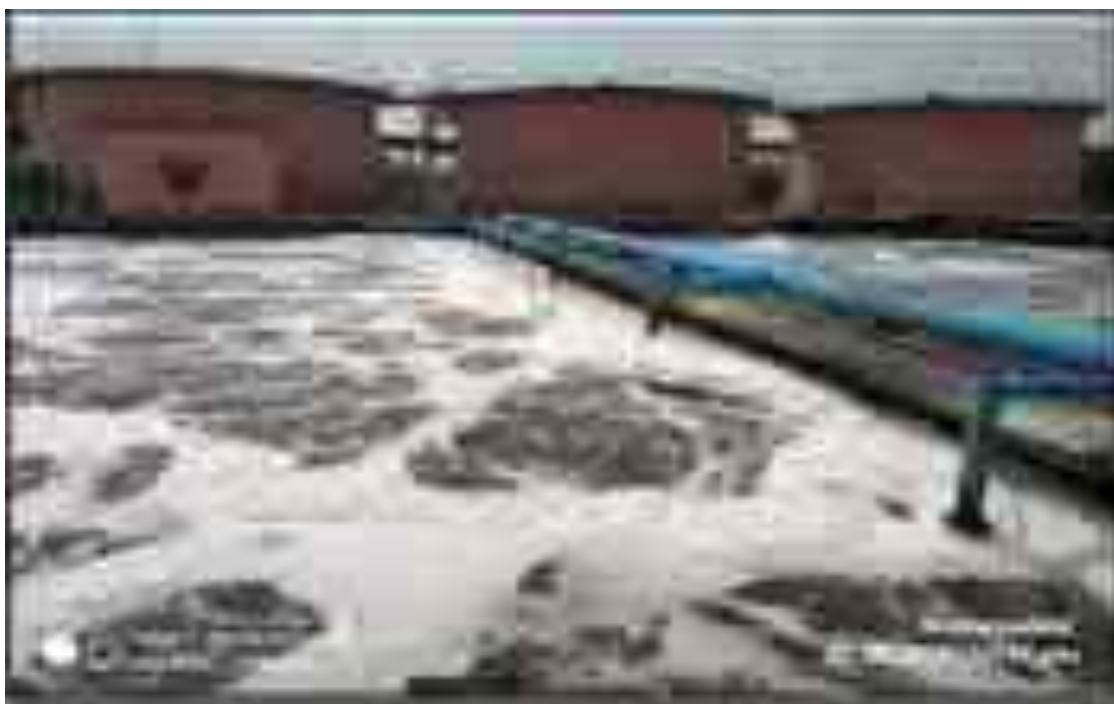
Aeration Tank – Commissioning work in progress
