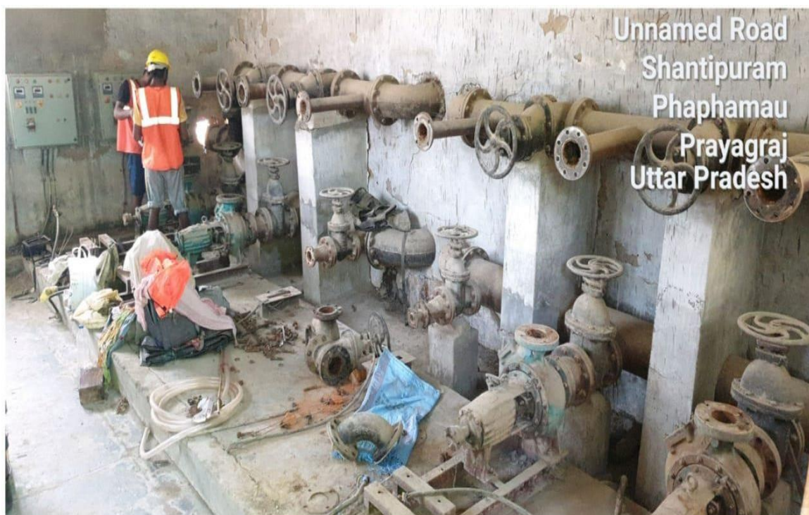
Pump House – Dismantling work in progress
