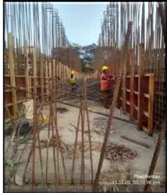
FCR tank – Shuttering work in progress
