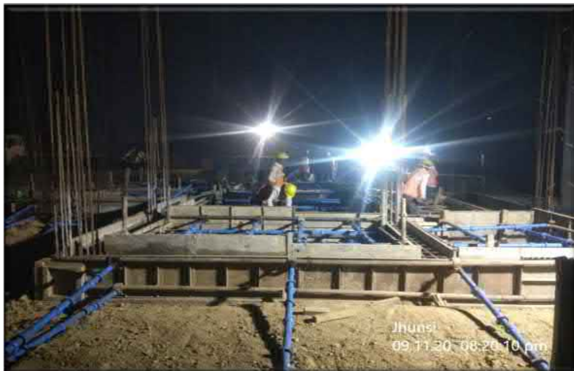
Staff Quarter – Shuttering work in progress
