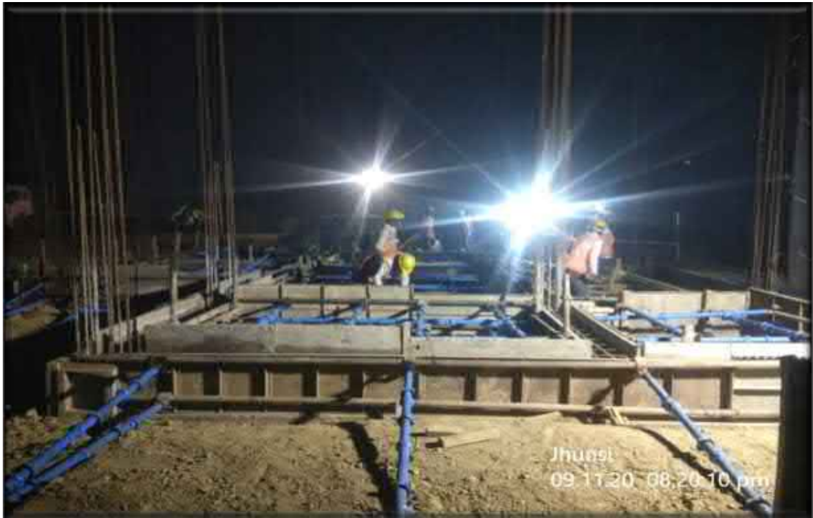
Staff Quarter - Wall footing reinforcement work in progress
