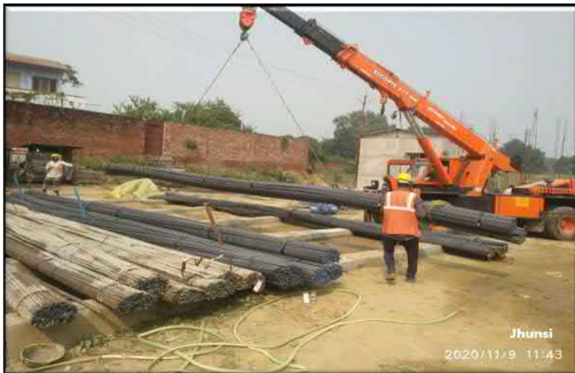
Stacking of rebar at Jhunsi STP
