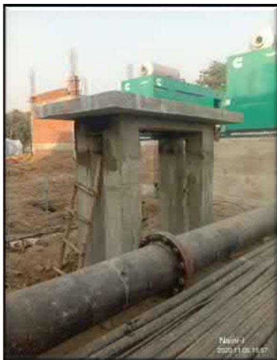
Oil tank – Foundation work completed
