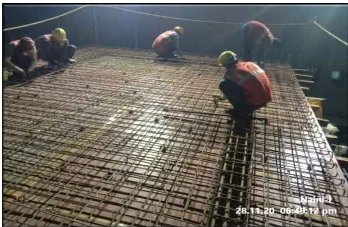
Wet mix filter - Building roof slab reinforcement work
