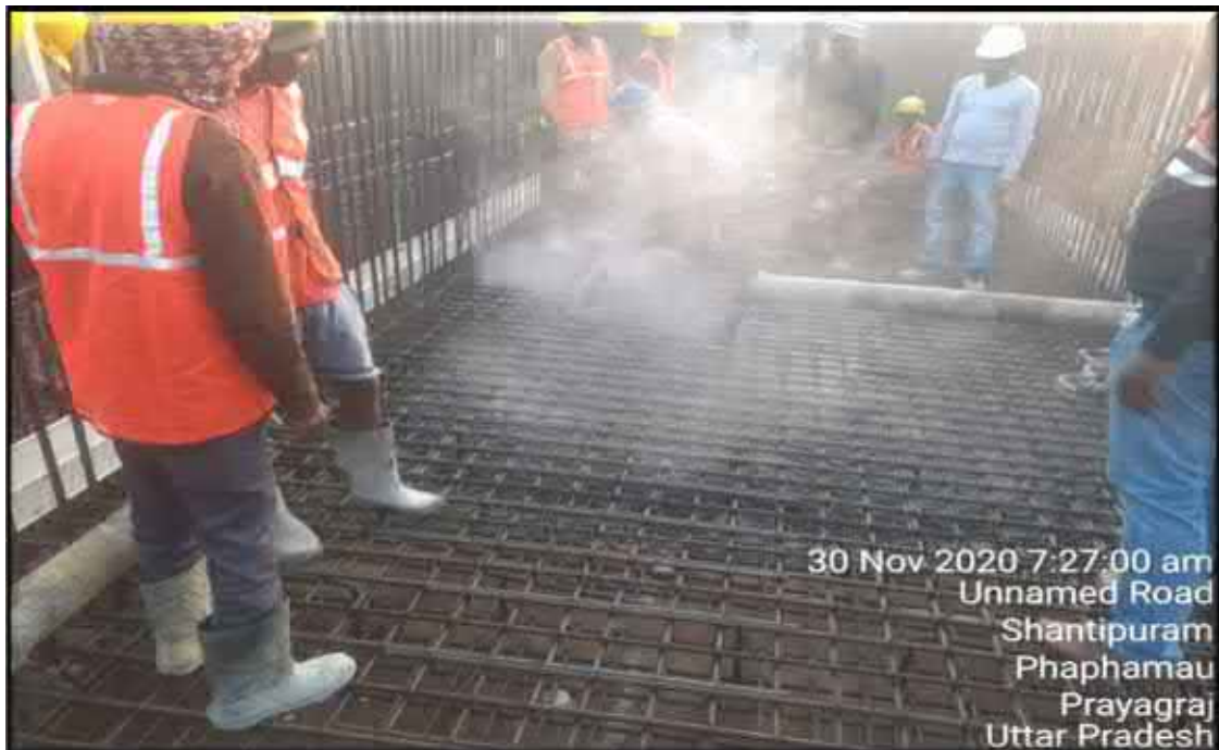
FCR tank – Raft Concreting work in progress
