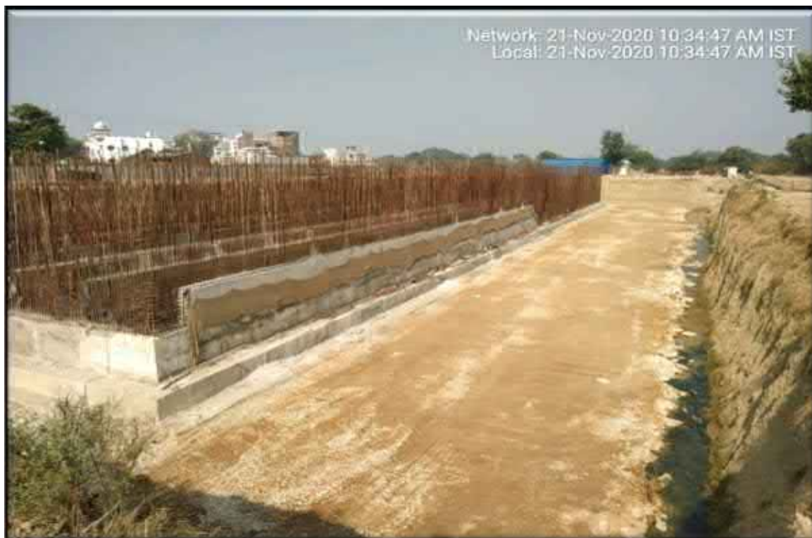
Tube settler tank - Soil compaction work in Progress
