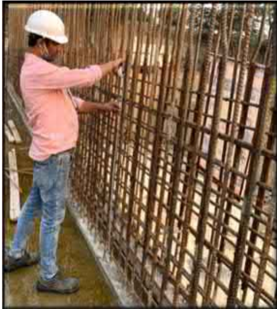
FCR tank - Lift wall reinforcement inspection by AECOM
