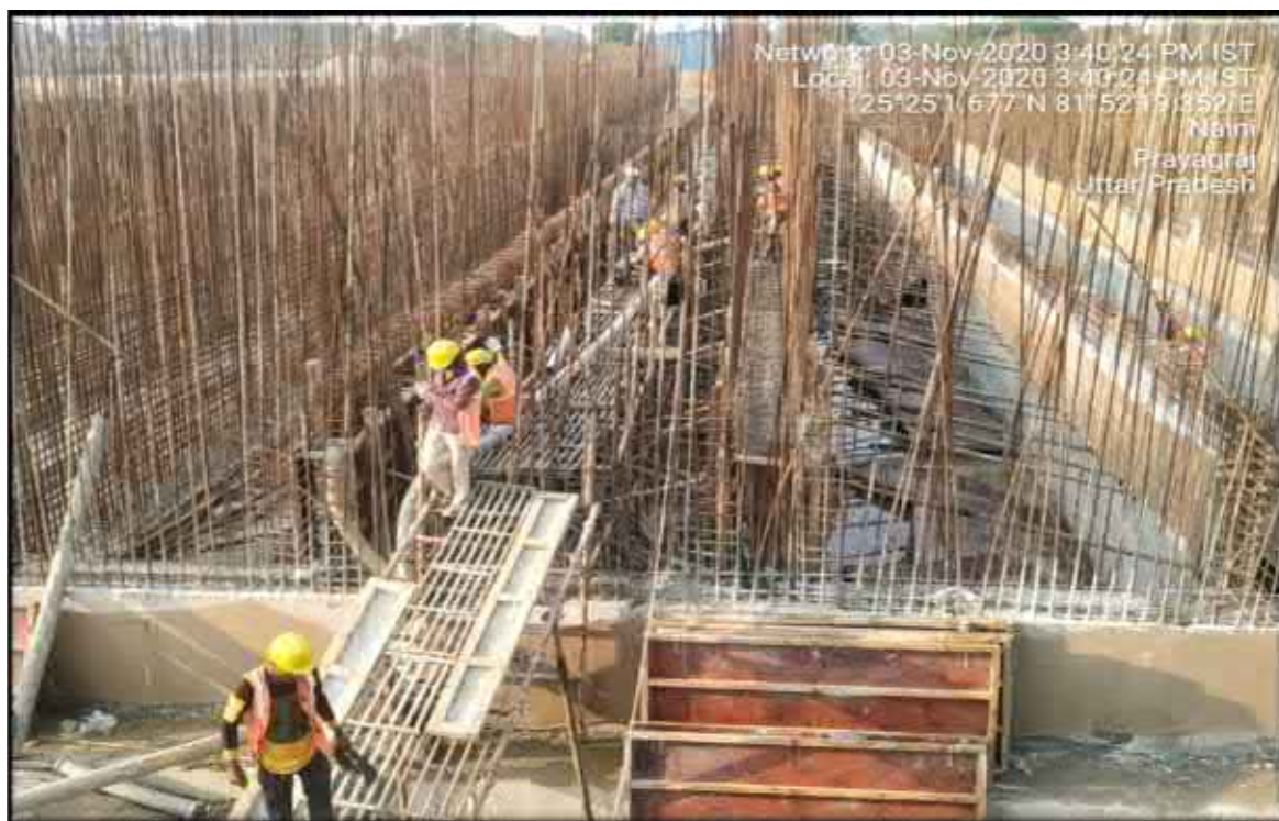
FCR tank –Shuttering work in progress
