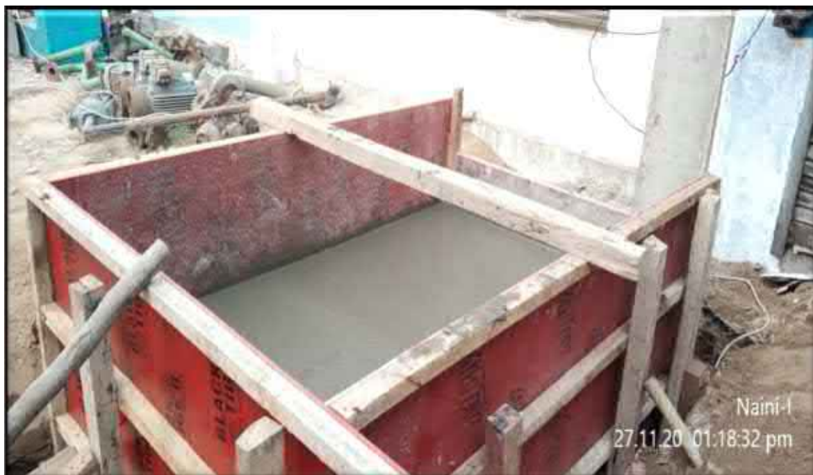
Hot water generator - Foundation casting work in progress
