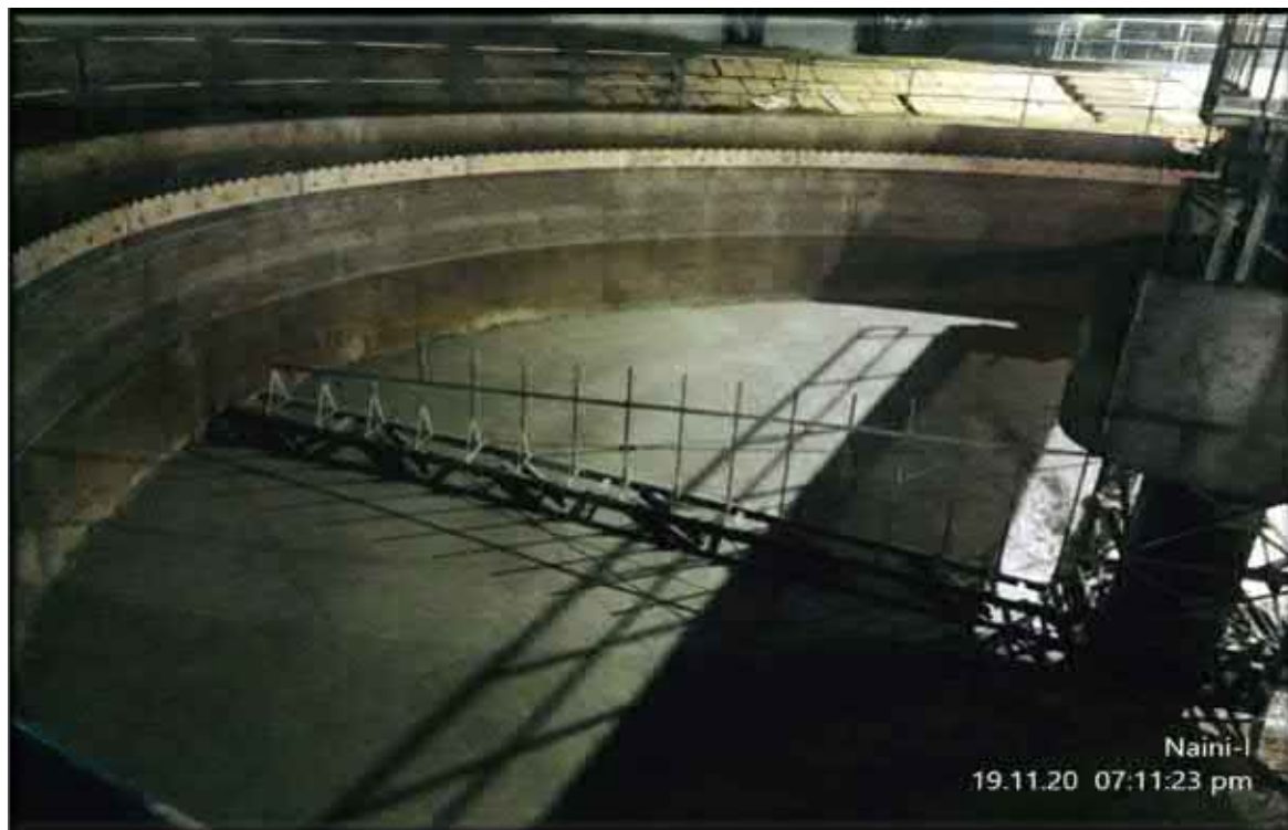
Thickener concrete screeding work completed
