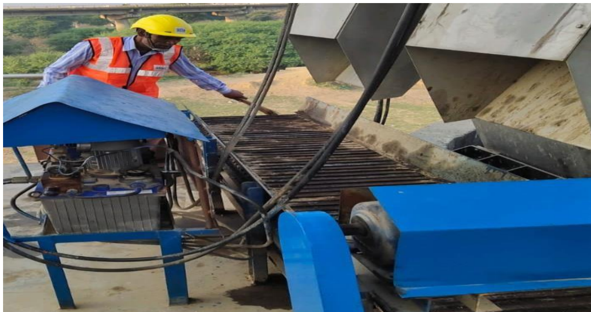
Mechanical screen – Cleaning & Lubrication work in progress
