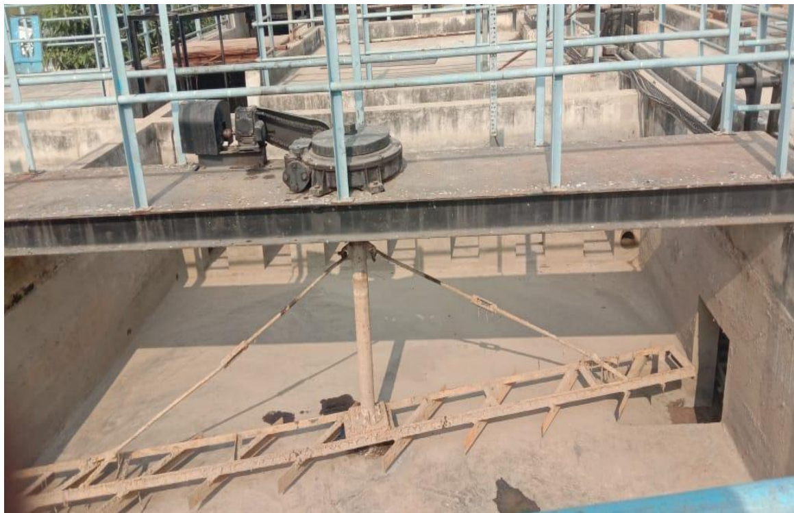
Grit Mechanism – Cleaning work in progress
