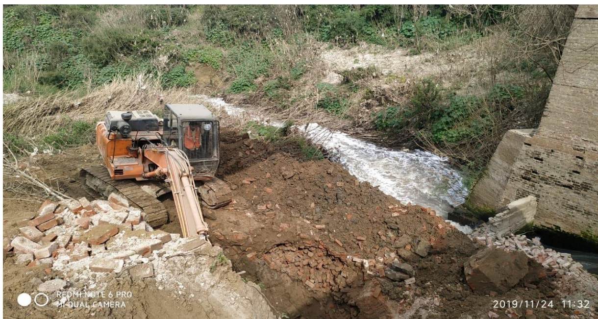
STP Outlet – Pillar excavation work in progress
