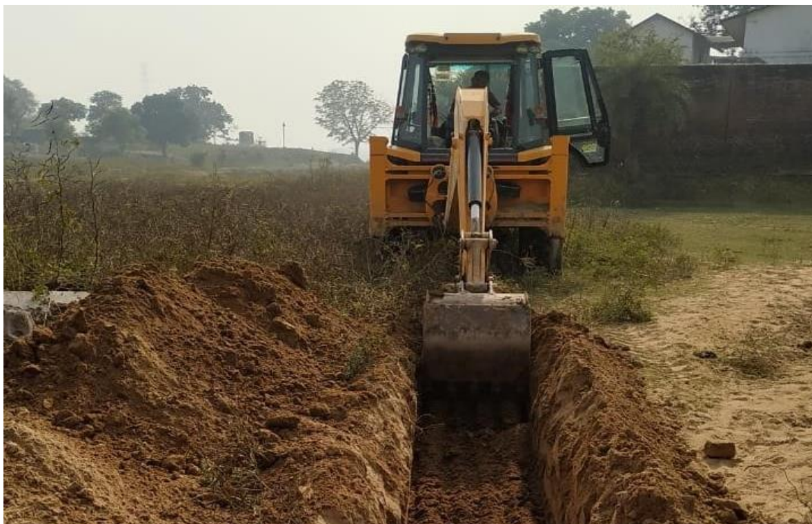
Boundary wall - Construction work in progress
