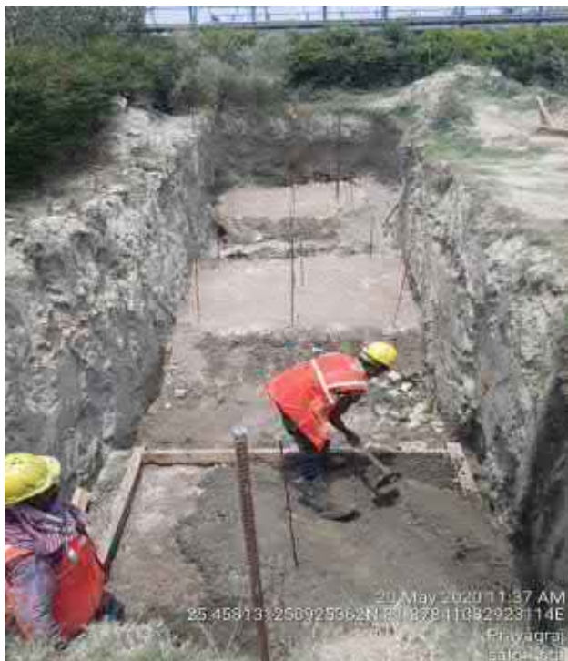
PLC Room – PCC work in progress
