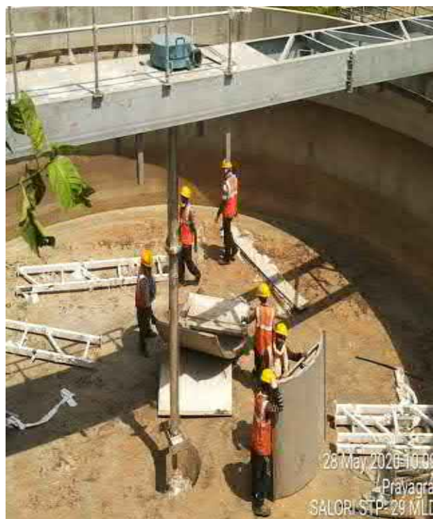
Clarifier – Thickner Erection
