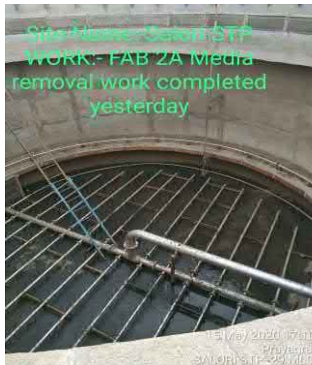
FAB Tank – Media removal work in progress
