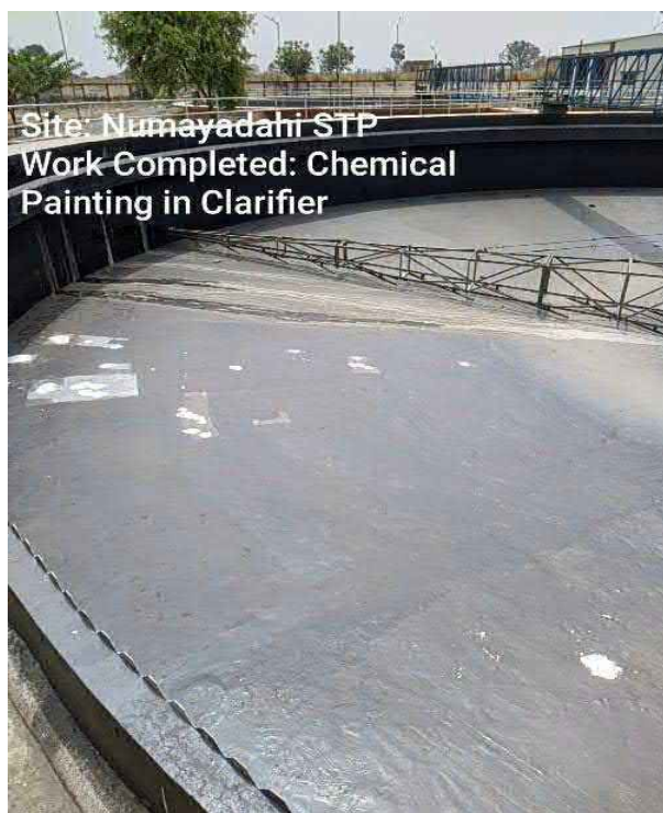
Clarifier - Surface finishing work in progress
