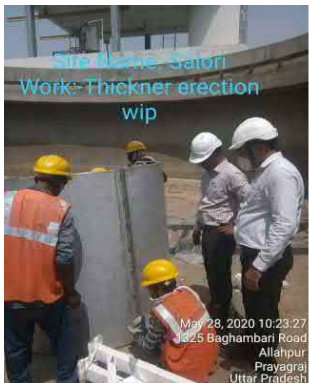
Clarifier – Thickner Erection
