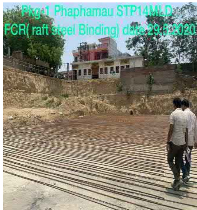
FCR – Raft steel binding work in Progress
