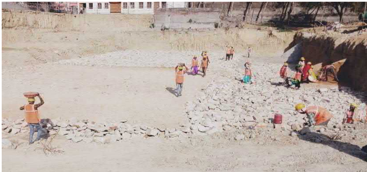
FCR – Boulder pitching work in progress
