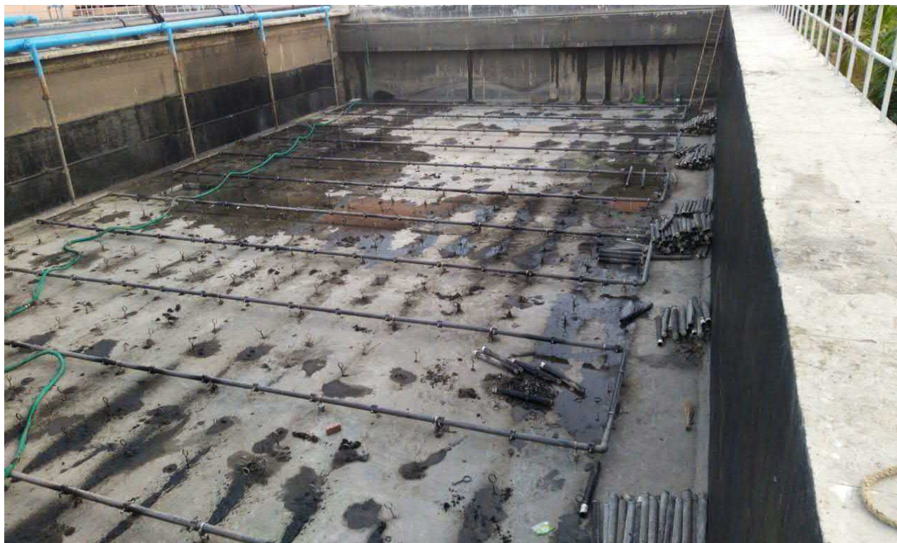
Aeration Tank (Diffuser) - Flushing work in progress
