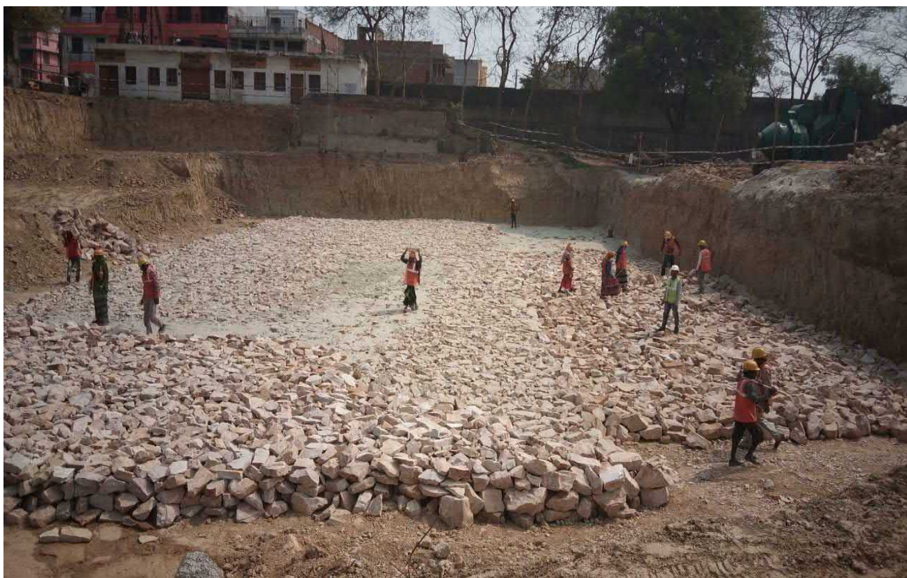
FCR – Boulder pitching work in progress
