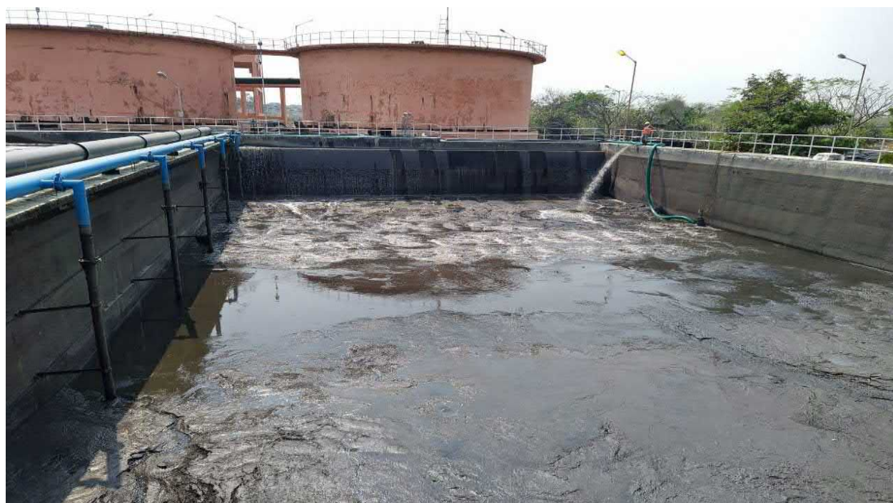
Aeration Tank – De sludging work in progress
