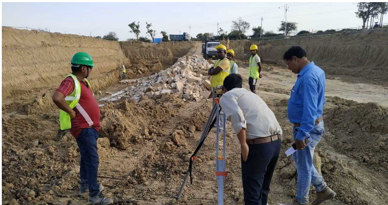
FCR – Excavation level checking by AECOM's engineer
