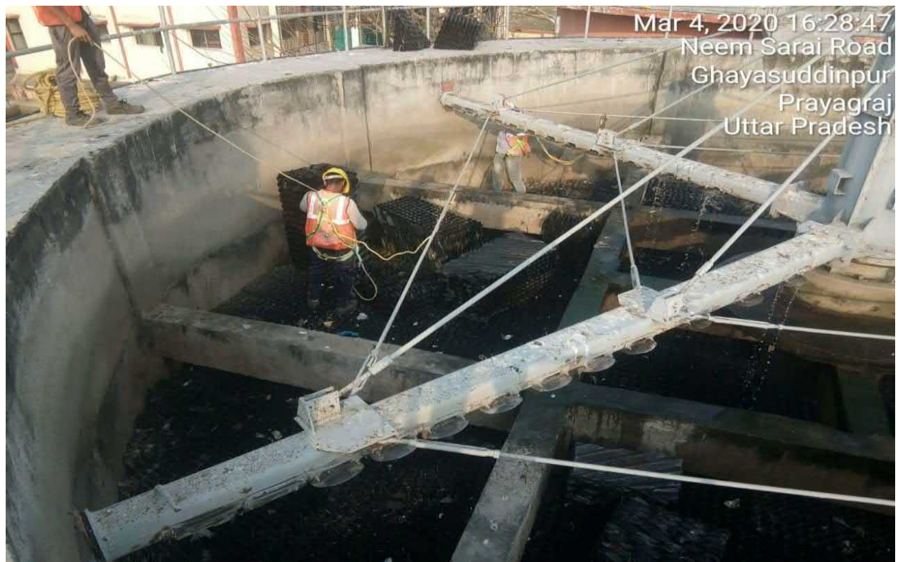
Bio Tower 2 –Media Replacement work in progress
