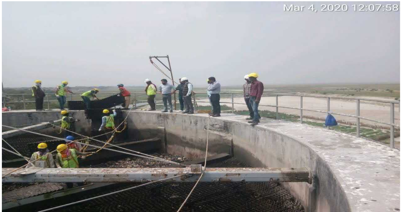
Bio Tower 2 –Media Replacement work in progress
