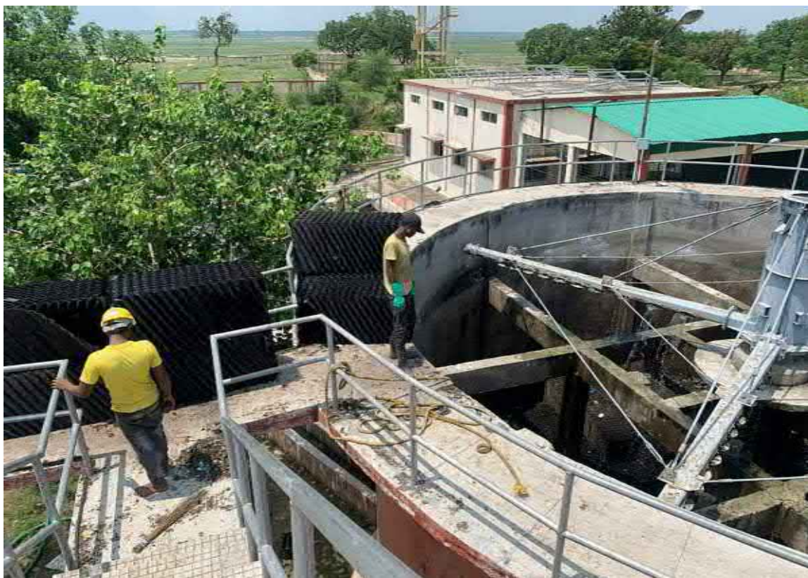
Bio Tower – Cleaning & Media Replacement work in progress
