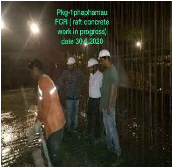
FCR – Raft concrete work in Progress
