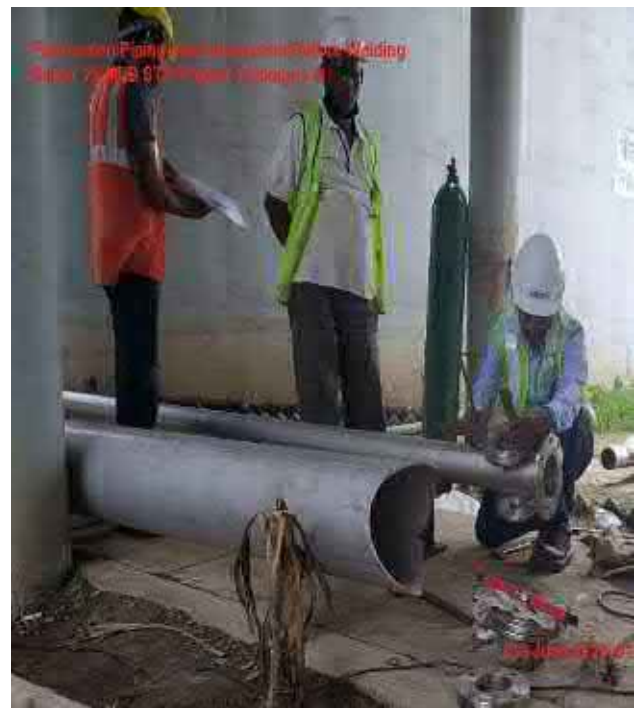
Fabrication joint inspection by AECOM Engineer after welding
