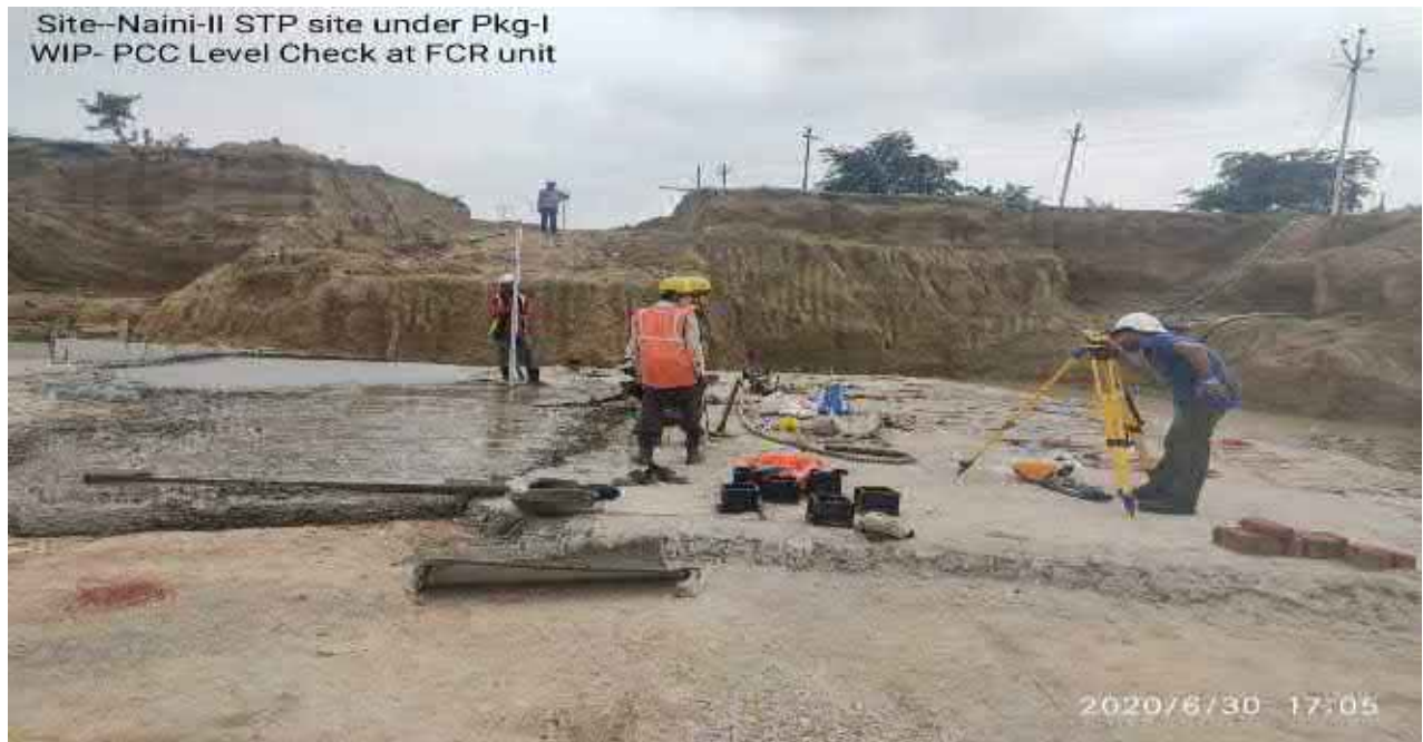
FCR – PCC Level check by Aecom Engineer
