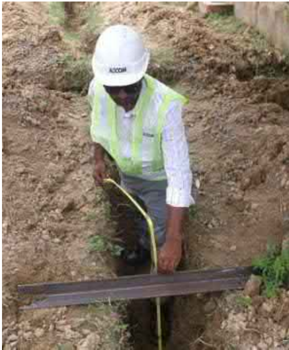
Cable trench inspection by Aecom
