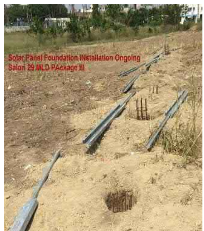
Solar Panel – Foundation work in progress
