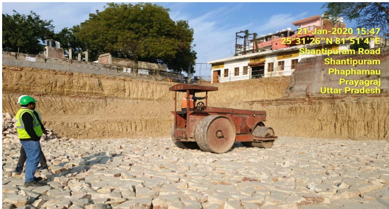
FCR – Boulder soling work in progress
