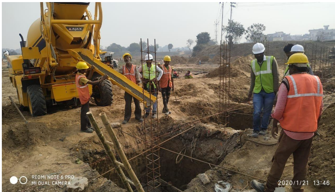
Boundary wall– Footing pouring work
