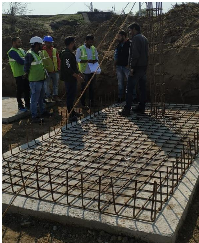
Staff Quarter – Reinforcement checked by UPJN official
