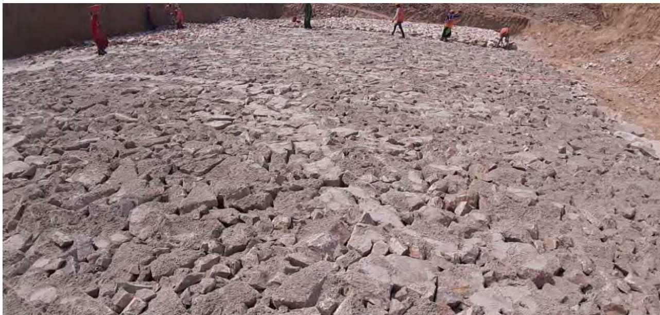
FCR – Boulder pitching work in progress
