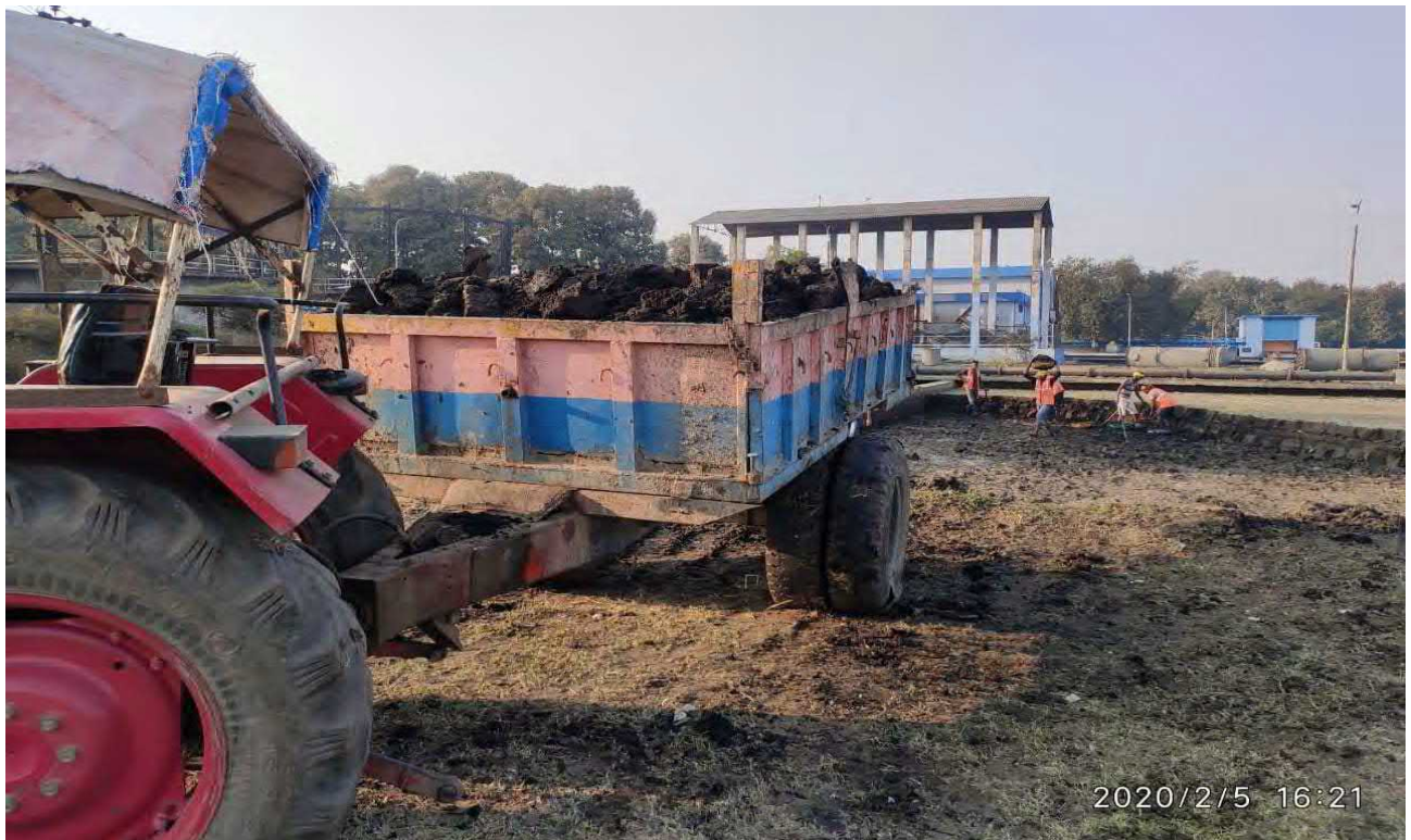
Sludge Drying Bed – Cleaning work in progress
