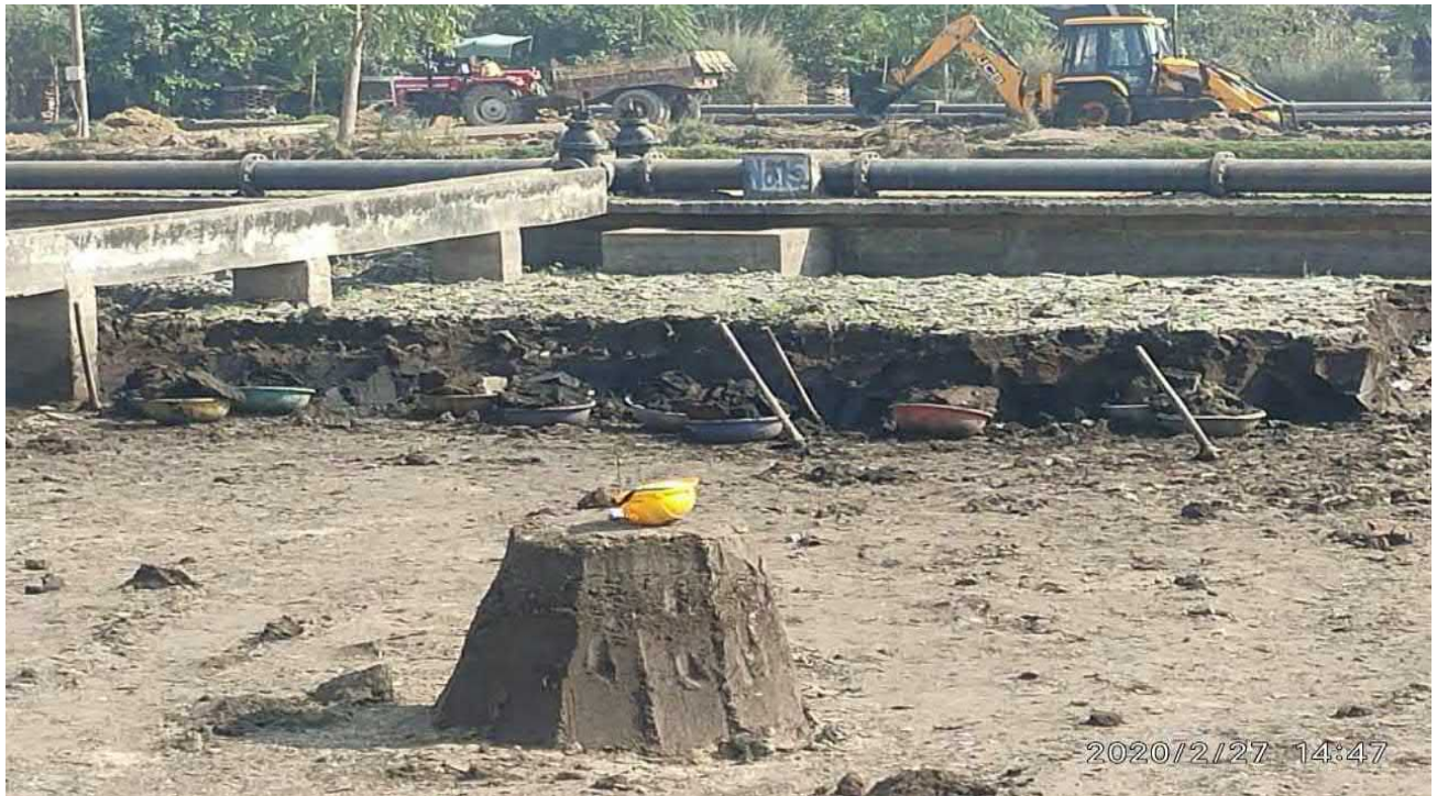
Sludge Drying Bed – Cleaning work in progress
