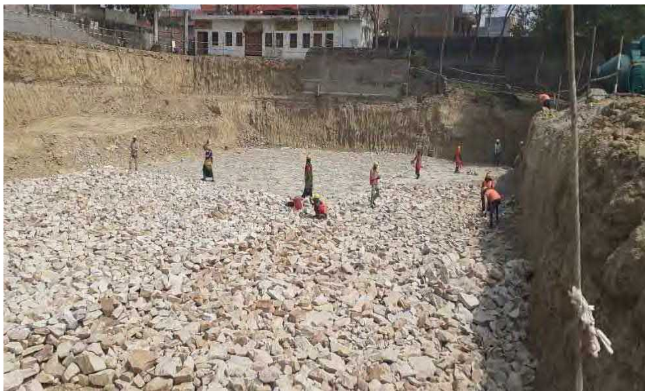
FCR – Boulder pitching work in progress
