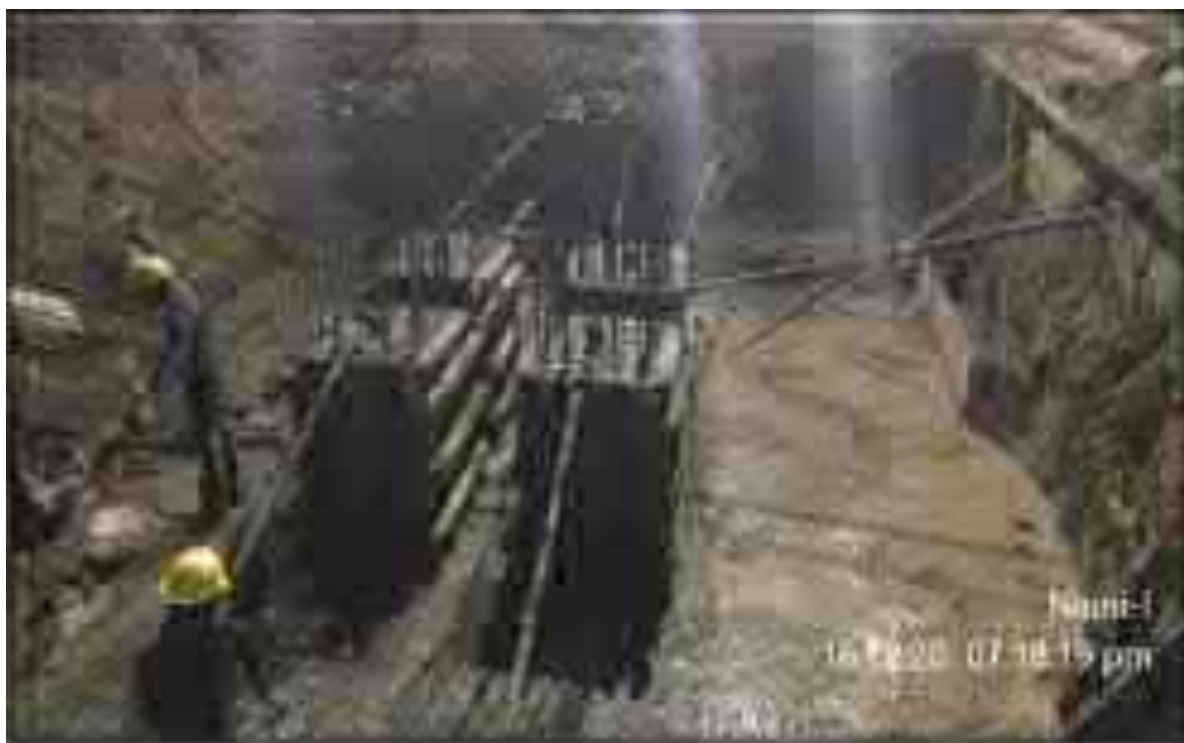
Chimney Foundation - Pedestal casting in progress
