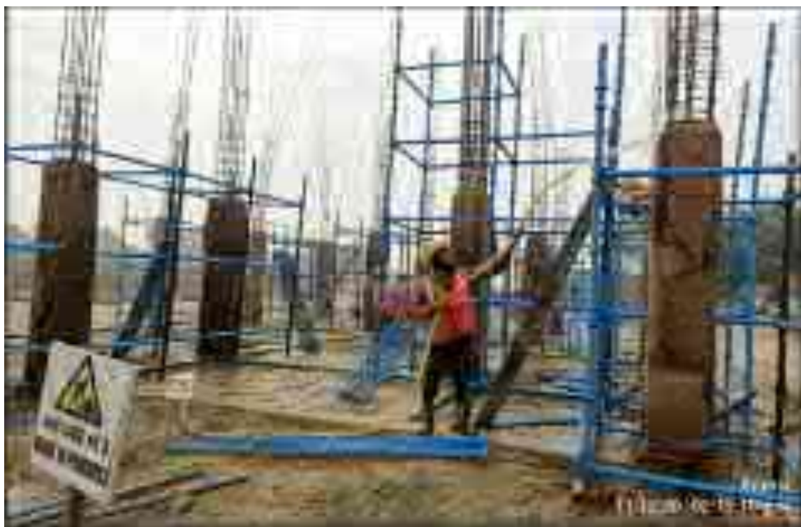
Staff Quarter – Column curing in progress
