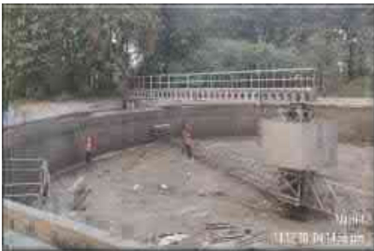
FST – Weir plate erection work in progress
