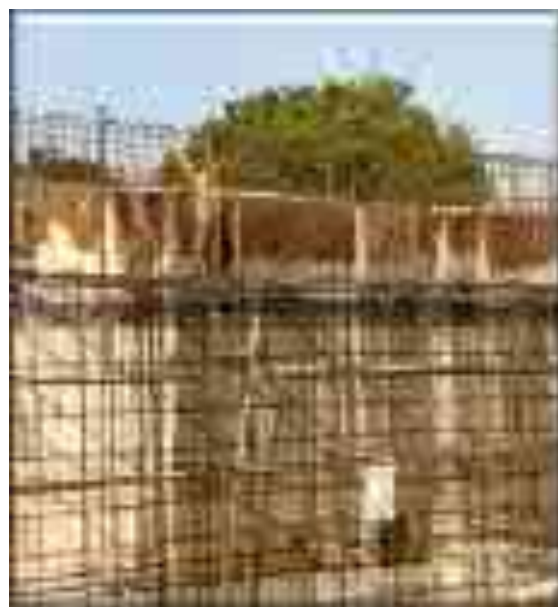
FCR tank – Lift wall curing under progress
