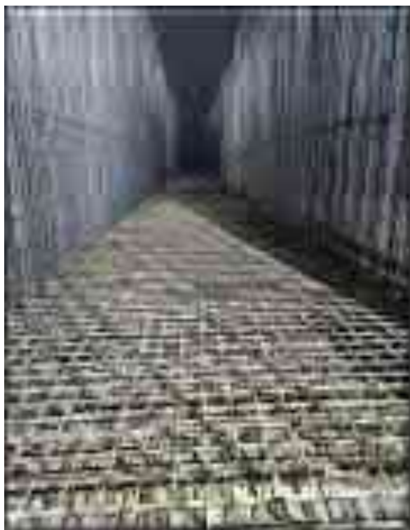
FCR Tank – Raft reinforcement completed
