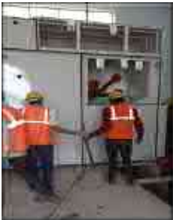
HT Panel - Installation work in progress
