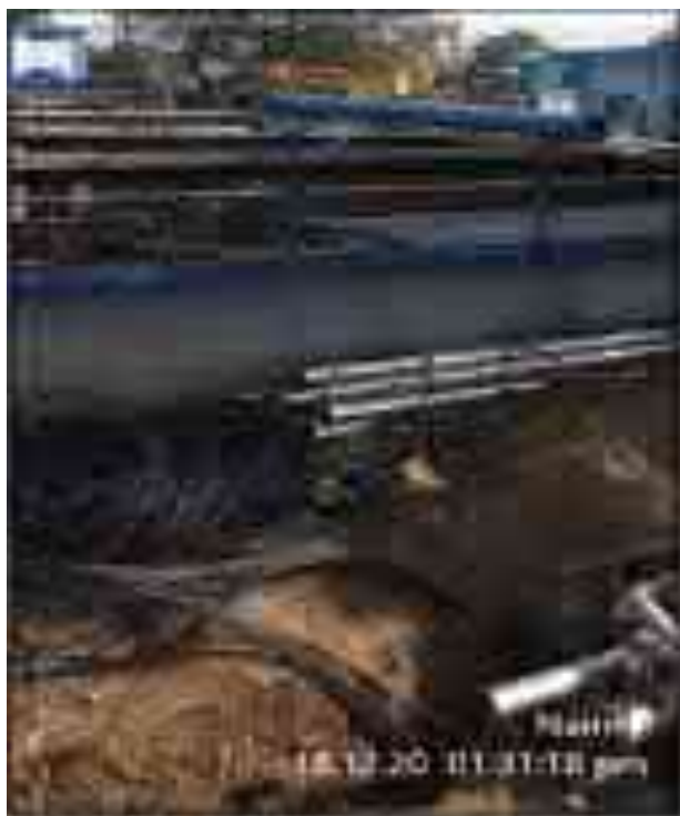
Aeration tank – Air piping dismantling work
