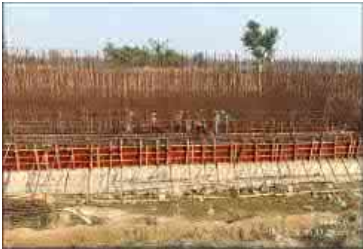
FCR tank –Lift wall concreting under progress
