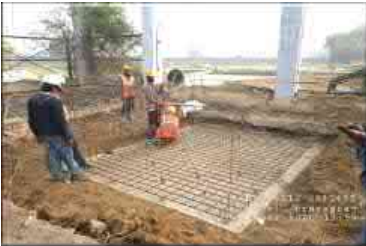
Dehumidifier – Steel binding work in progress
