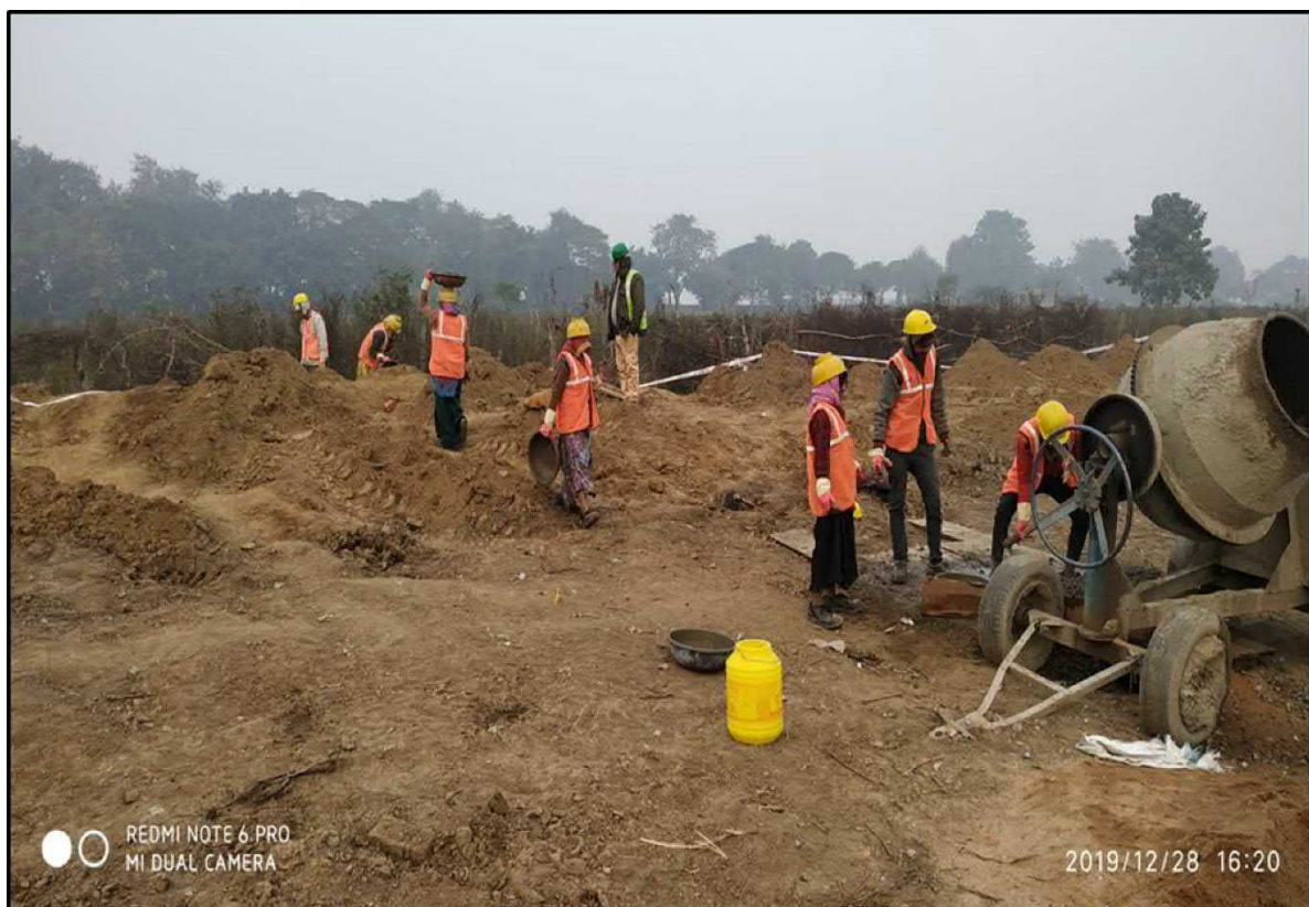
FCR tank – Excavation work in progress
