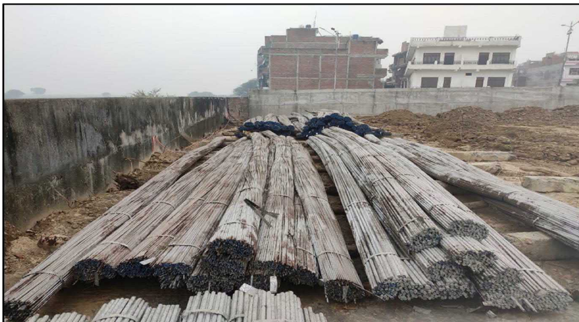
TMT steel received at site
