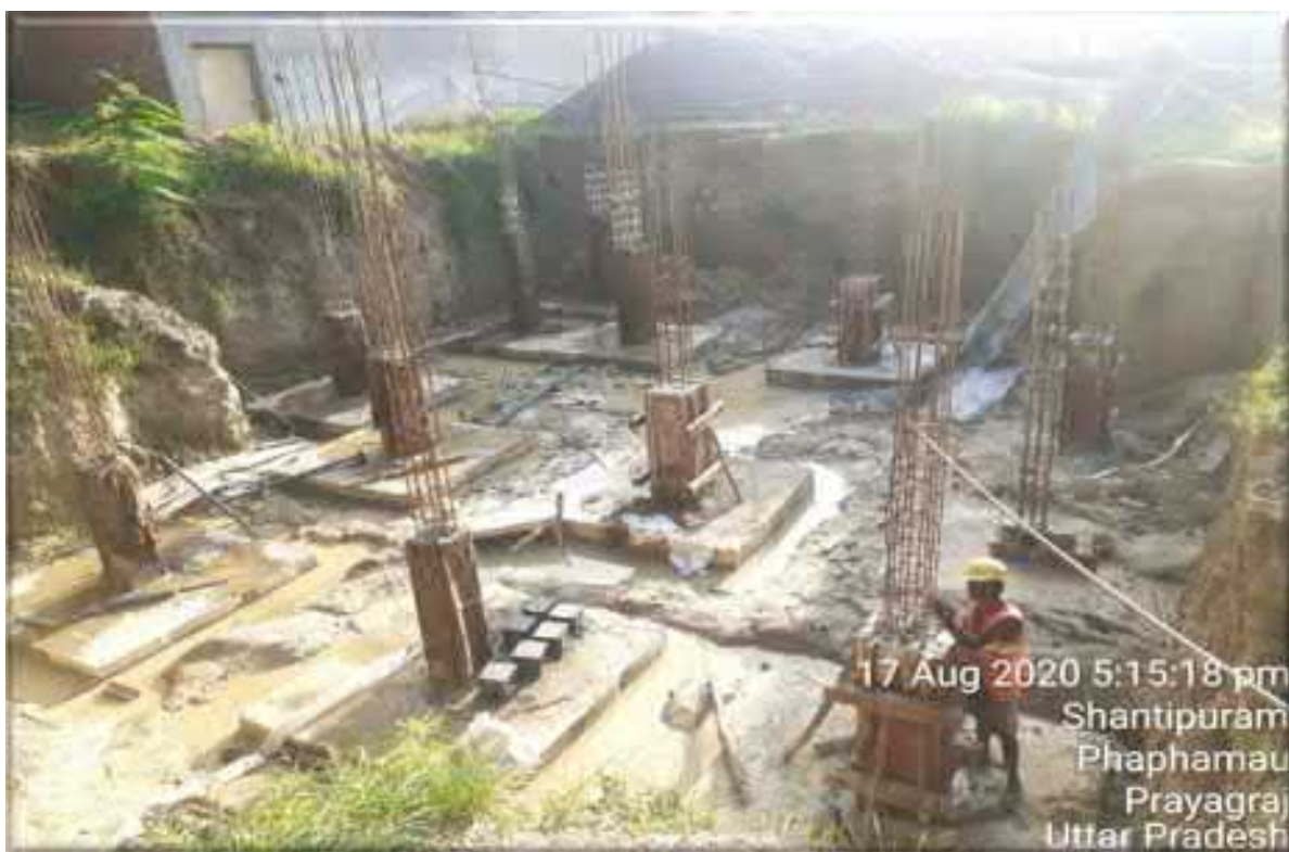
FCR tank - Staff quarter column shuttering work
