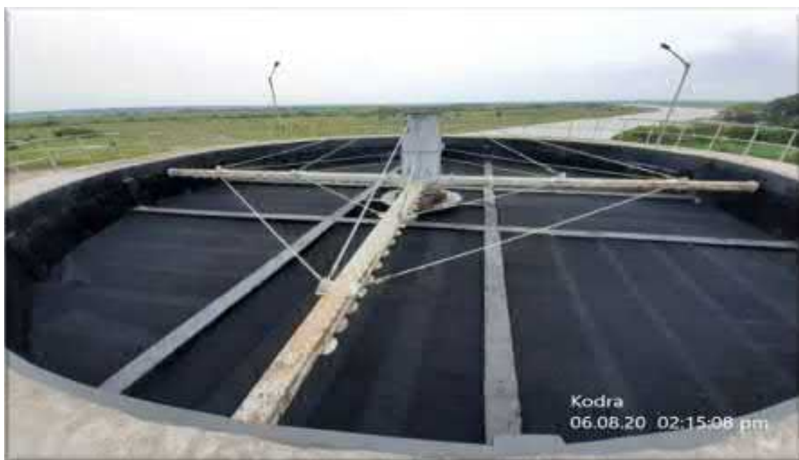
Installation of chicken mesh in Bio tower
