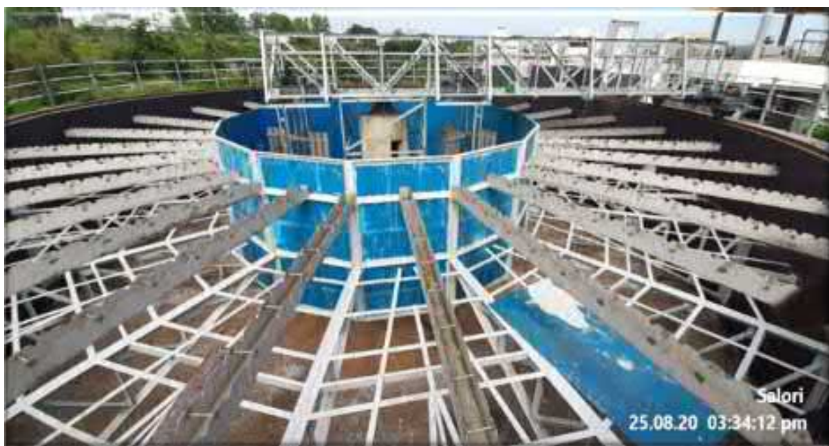
Clarissettler No. 2 - Bridge & launder erection completed
