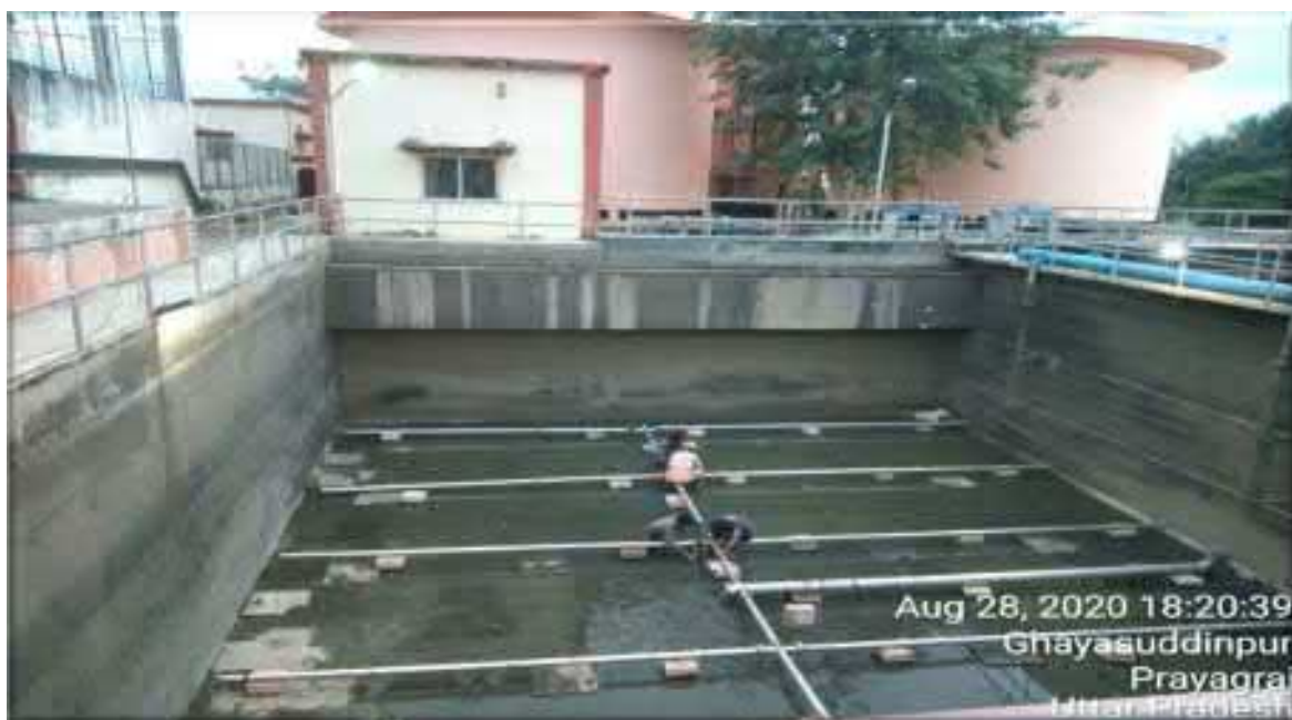
SS pipe installation in Aeration tank
