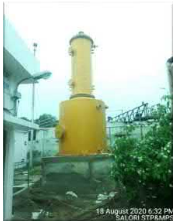
Chlorination absorption tower assembly work completed
