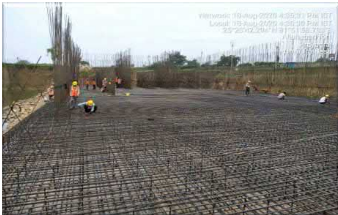
FCR tank - Reinforcement work in progress
