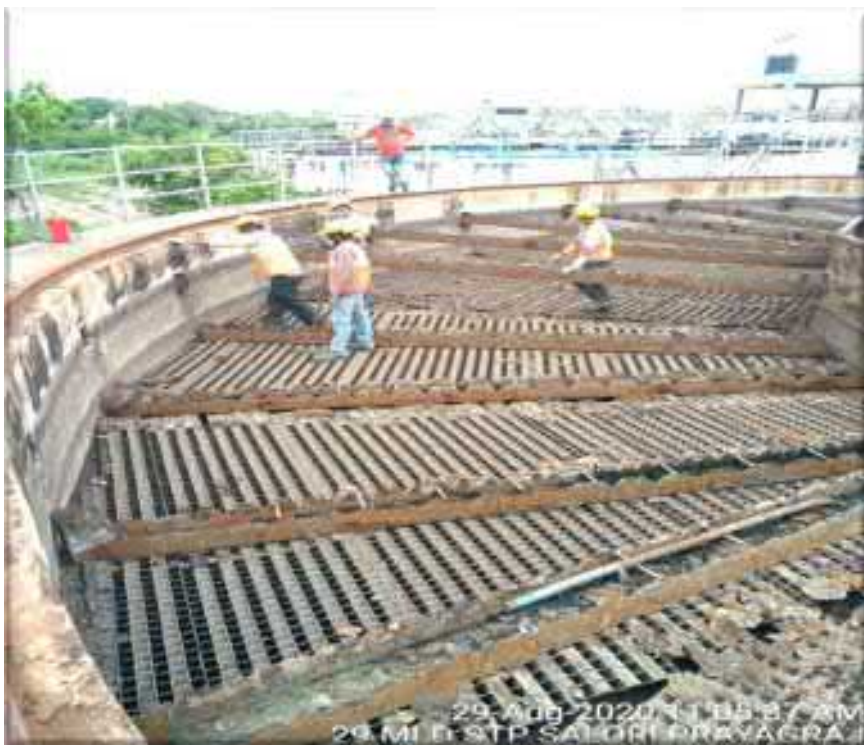
Clarissettler No. 1 - Dismantling work in progress
