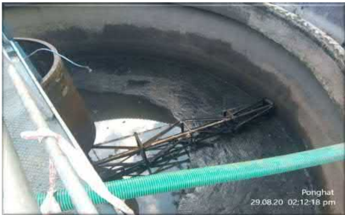
Desludging of thickener completed
