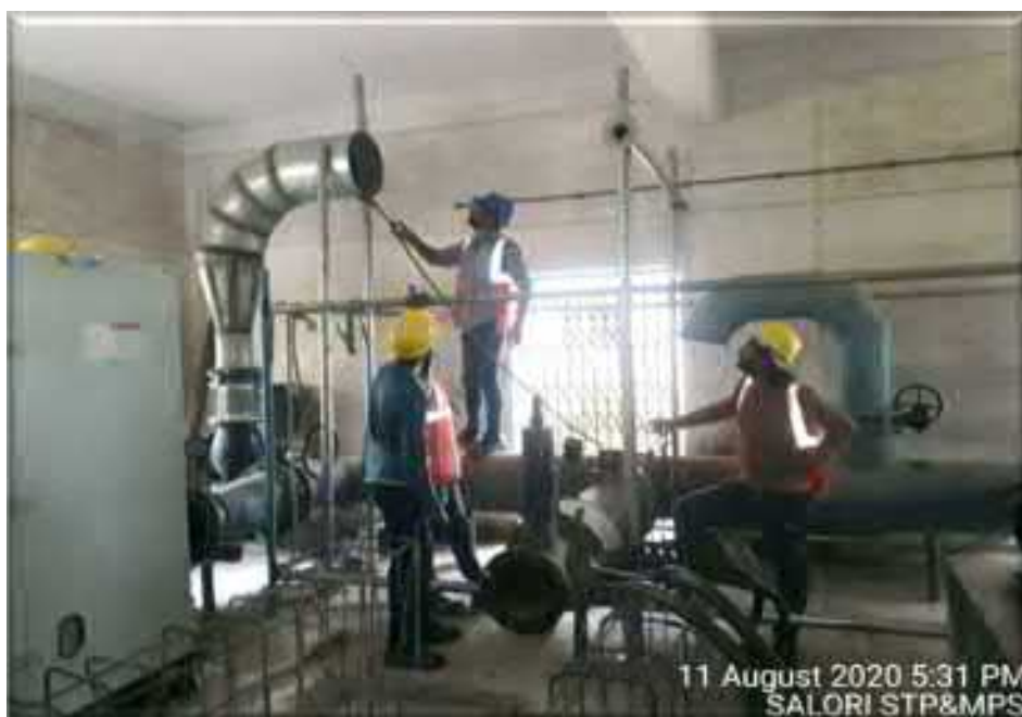
Erection of blower header
