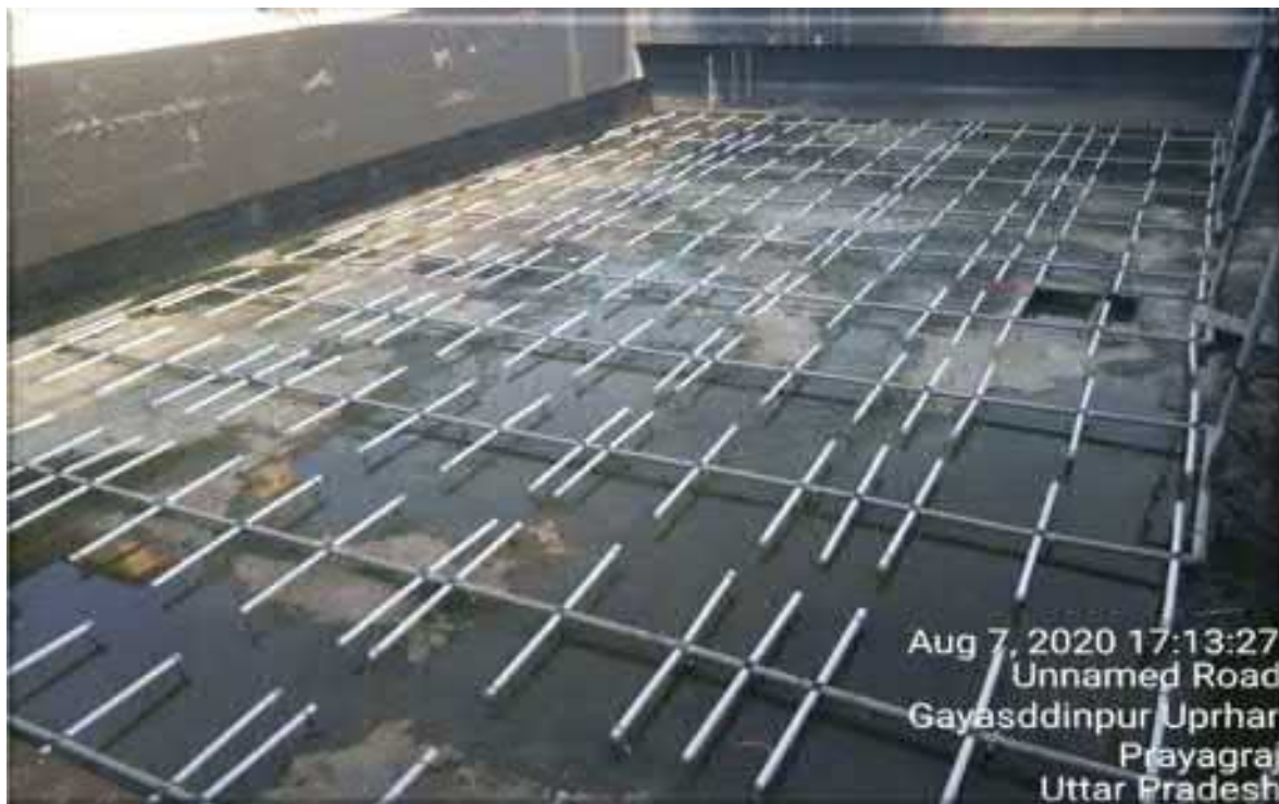
Erection of diffuser completed in aeration tank
