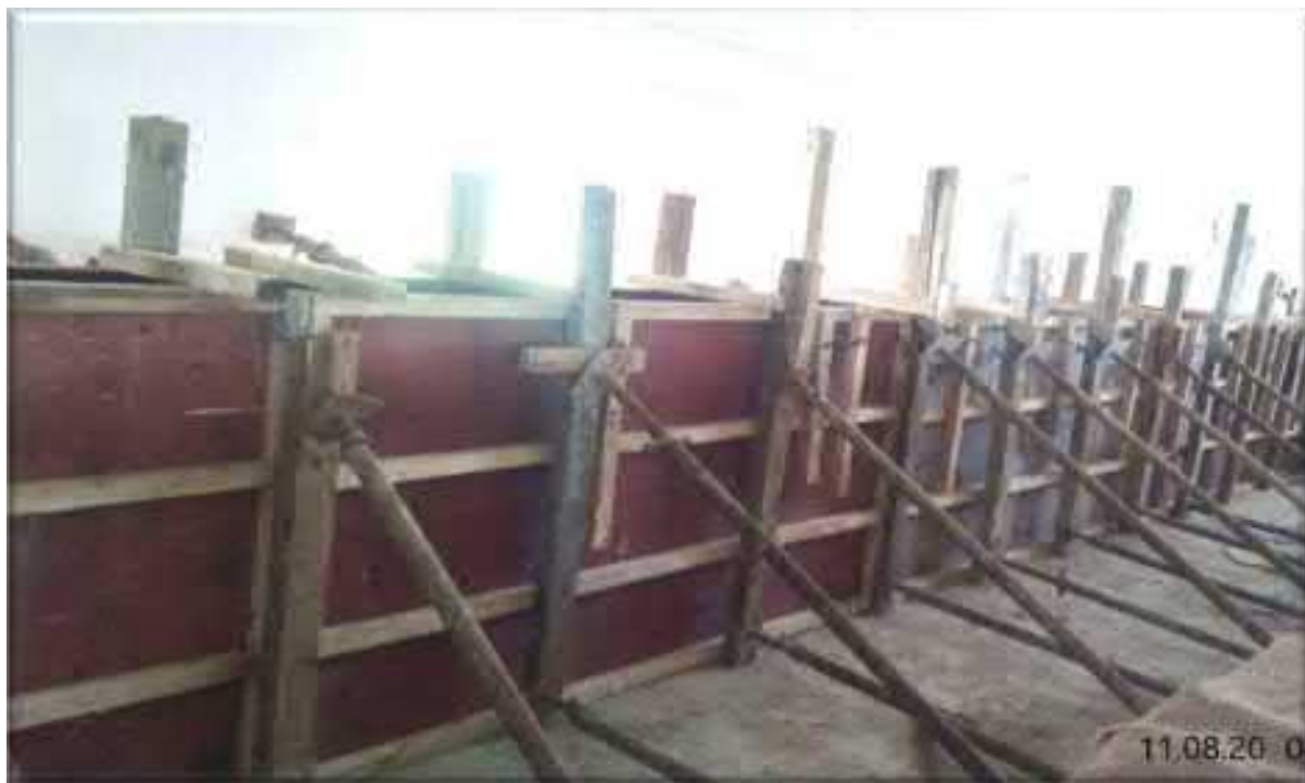
MEP room - Shuttering work in progress
