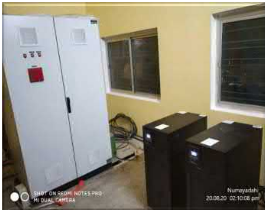
PLC panel & UPS charger installation work completed
