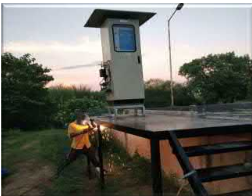
At Outlet point - Analyzer erection completed & fabrication of frame in progress
