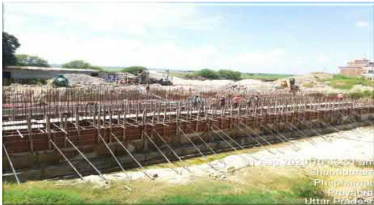
FCR tank - Shuttering work in progress
