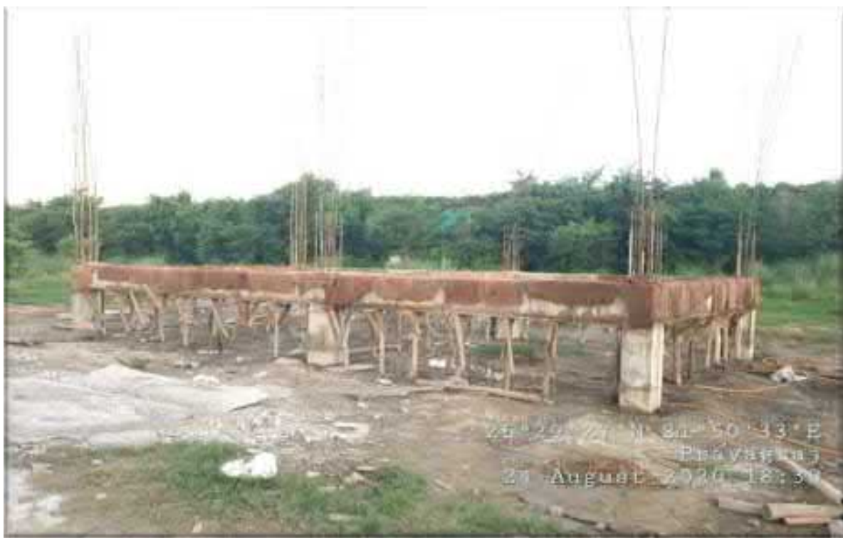
Battery room – Curing at RCC column and tie beam in progress
