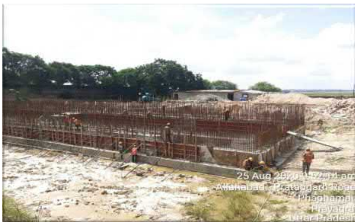
FCR tank - Lift wall shuttering work in progress
