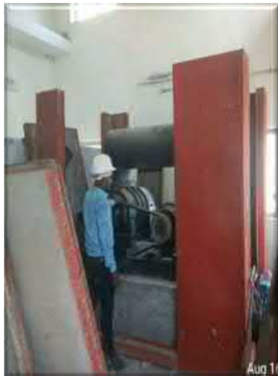
Dismantling of Blower No. 3
