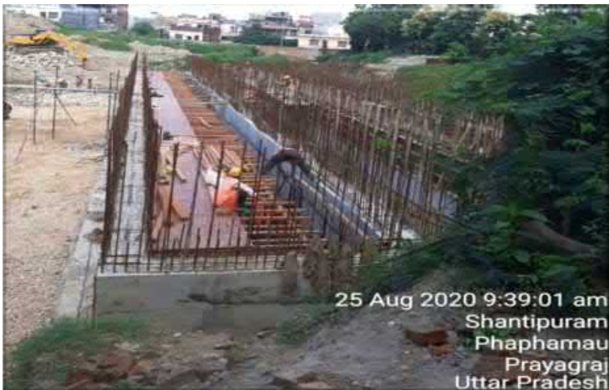
FCR tank - Shuttering work in progress
