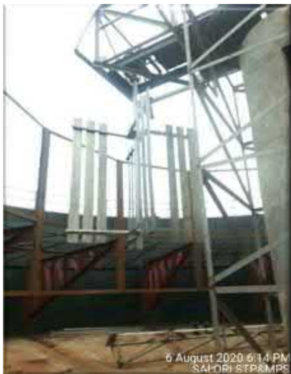
Flocculator assembly installation completed
