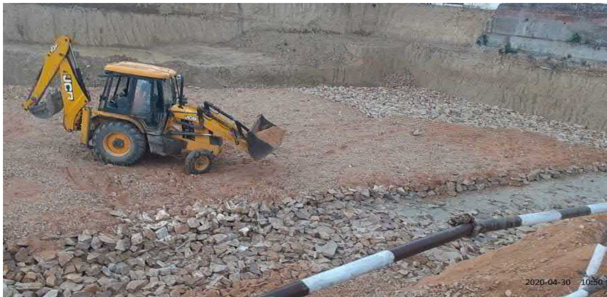
FCR – Boulder pitching & sand filling work in progress
