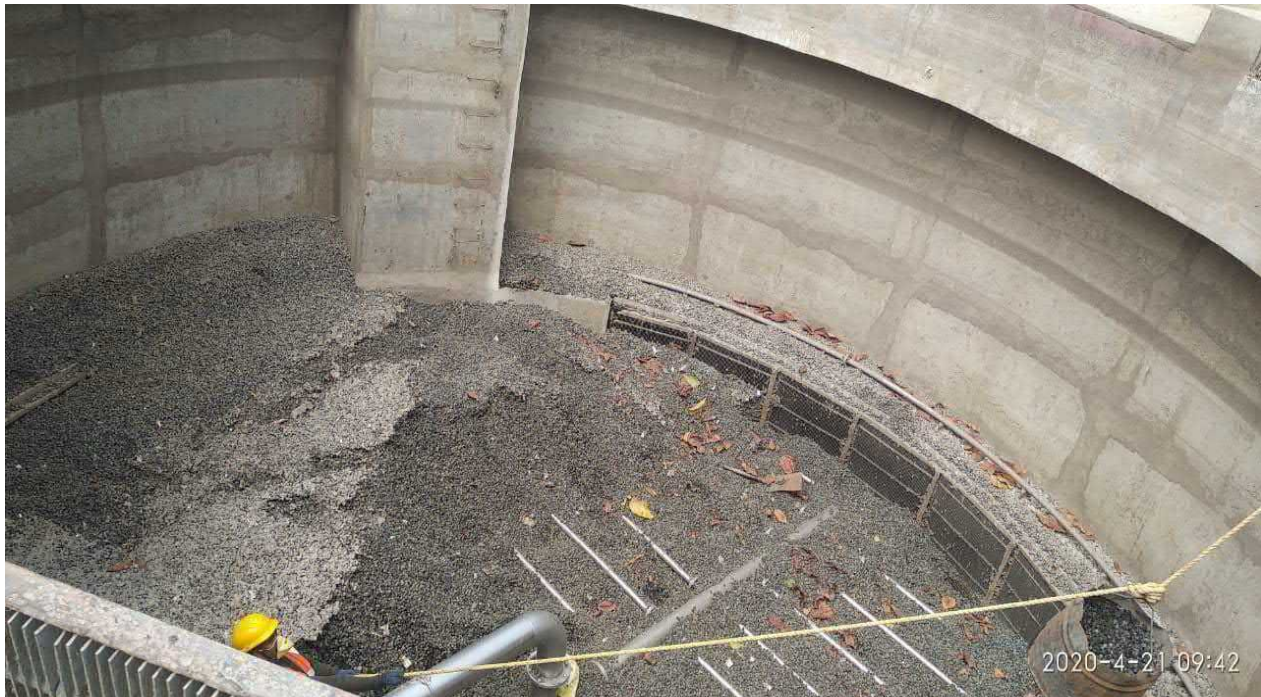
FAB Reactor – FAB media removal work in progress
