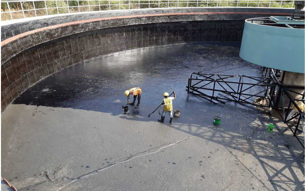
Secondary Clarifier - Epoxy paint work in progress
