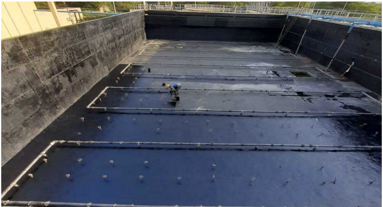
Aeration Tank - Epoxy paint work in progress
