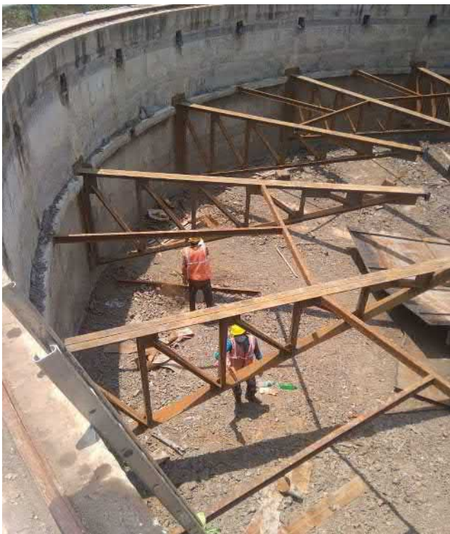
FAB Reactor – FAB media removal work in progress
