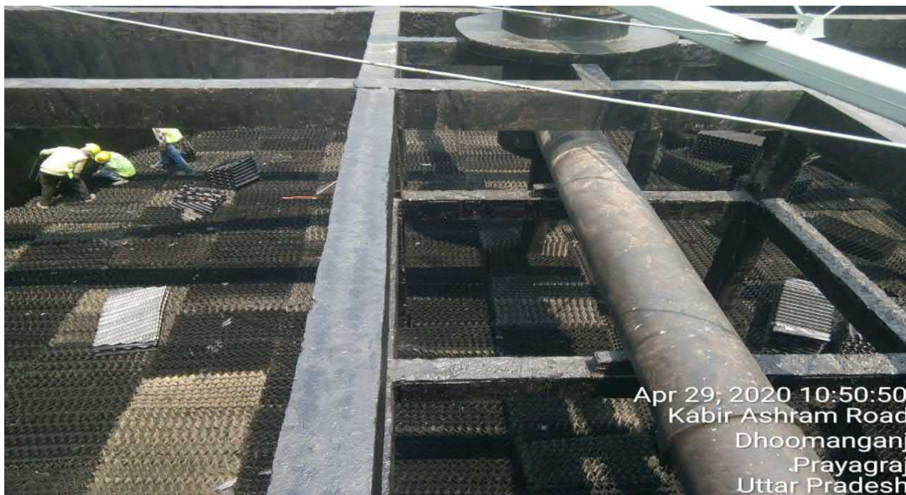
Bio Tower 2 – Cleaning work in progress
