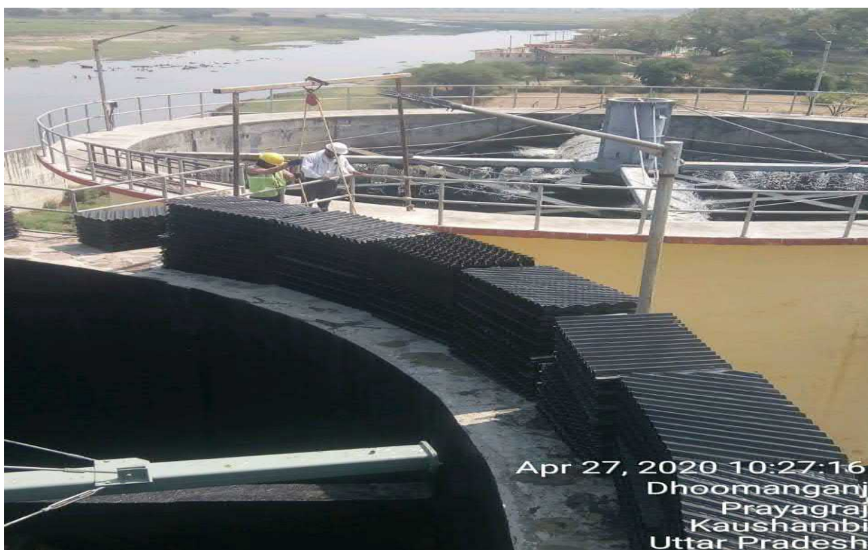
Bio Tower 2 –Media Replacement work in progress
